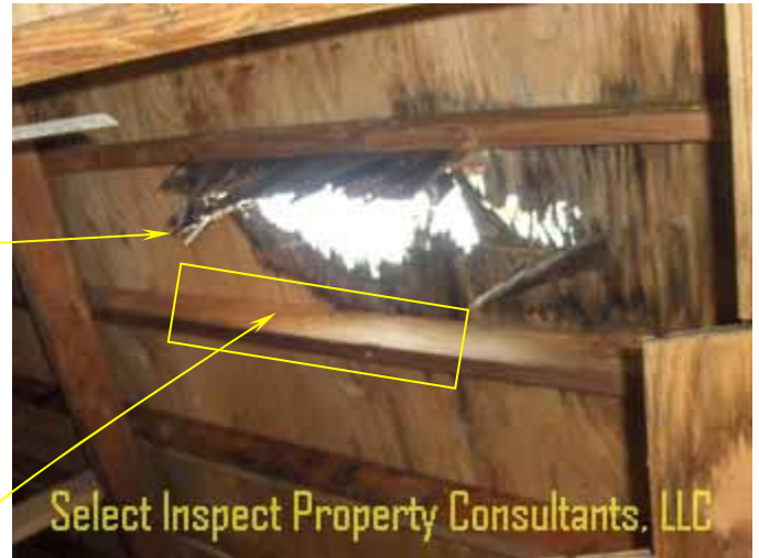
↑ attic of detached garage
