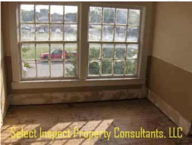
↑ window(s) lower than 24" interior & higher than 72" exterior
