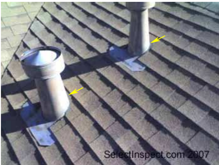
↑ tar repair at flues- example
