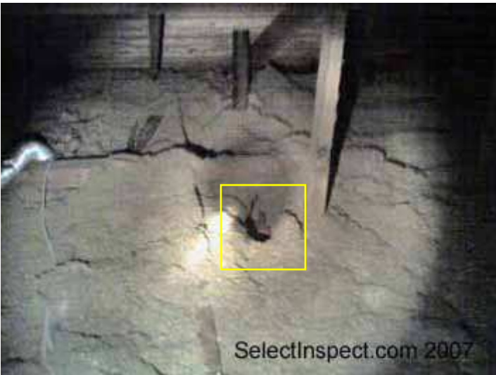
↑ amiss insulation at furdown- example
