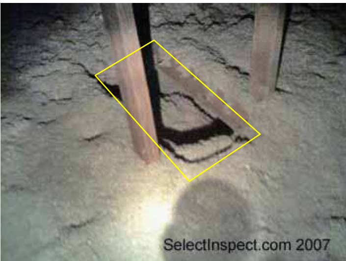
↑ amiss insulation at furdown- example 2
