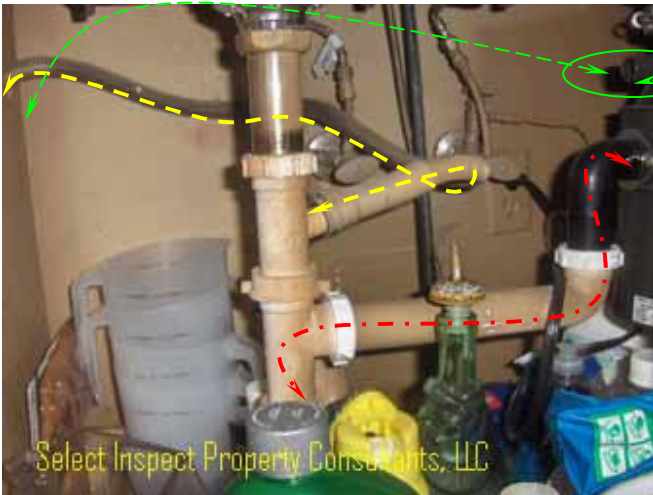
↑ dishwasher drain was incorrect & long route from disposal to drain trap
