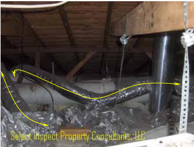
↑ inadequate support of air ducting; example
