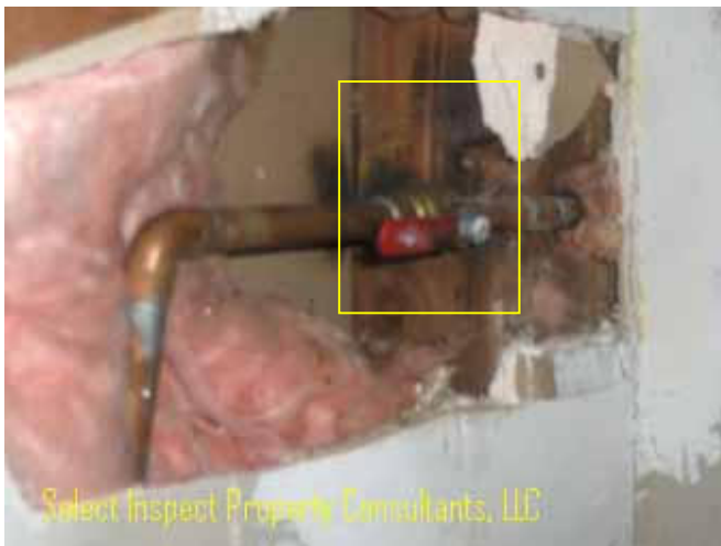
↑ stud under south bathroom sink notched at 28.57%; did not appear to be load bearing at this location; monitor.
