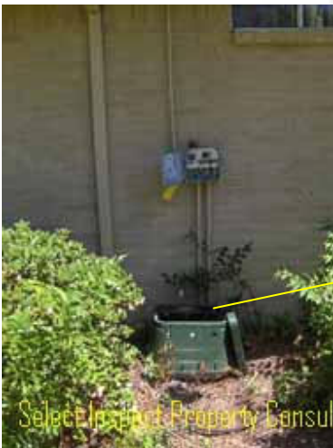
↑ septic agitation pump box
