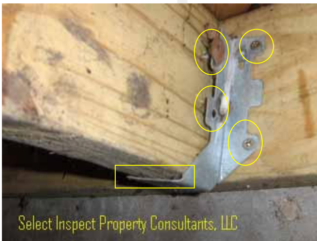
↑ below decking- incorrect fasteners & unworkmanlike joist hanger installation example
