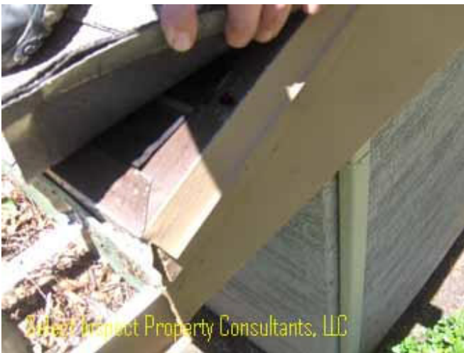
↑ example-unworkmanlike drip edge/felt; corners should have no gaps; rake (diagonal) edge & roof felt should be atop the eave (lower) edge flashing; roof underlayment should be under rake flashing
