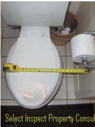
↑ toilet at east bathroom & master did not have required clearance
