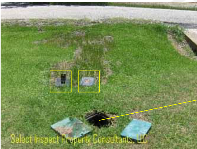
↑ water meter on left; irrigation meter on right
