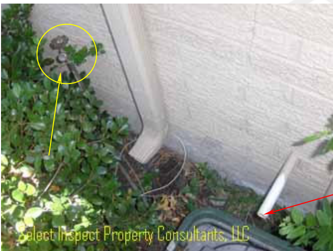
↑ inoperable exterior faucet(s) & improper termination (& wrong pipe material) of south water heater temperature/pressure relief & missing block/extension at gutter down-spout
