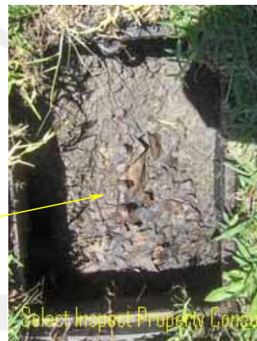
↑ Shut-off-valves require 3" clearance from soil; irrigation anti-siphon; corrosion; damaged lid
