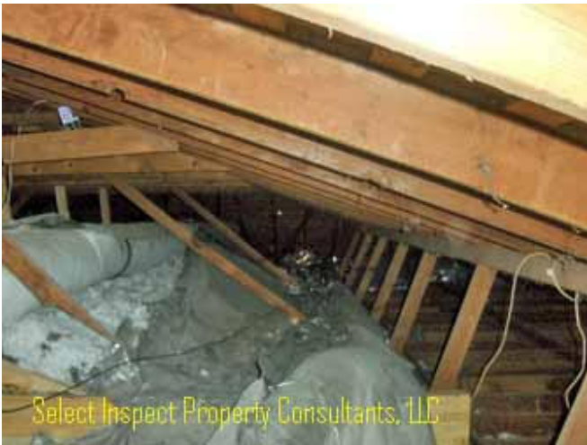
↑ southwest & south attic not readily accessible
