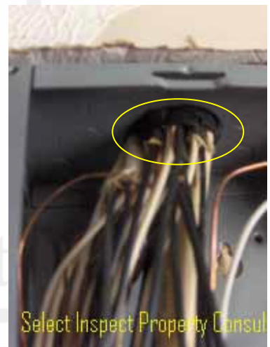
↑ deficient bushing at electrical cabinet
