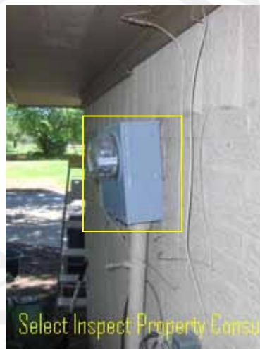
↑ inadequately secured electrical meter
