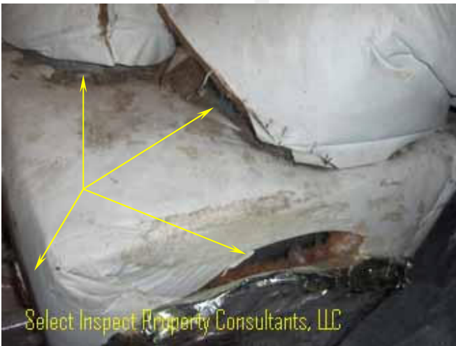
↑ energy loss at air ducting; inadequate insulation & seals; example at plenum/manifold
