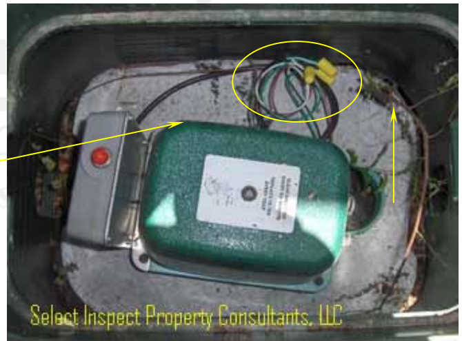
↑ foliage & missing electrical junction box
