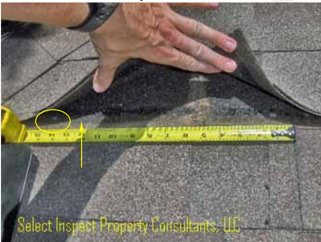
↑ improper nailing discovered at random shingles; example- should be 1" & 12" from each end, this one is 1" & 14"- Immediate corrective needs were not discovered
