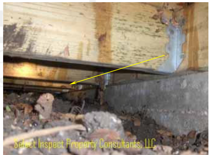
↑ all visible joist hangers under the deck were incorrect. & low deck/high soil can limit ventilation & may eventually be prone to fungus
