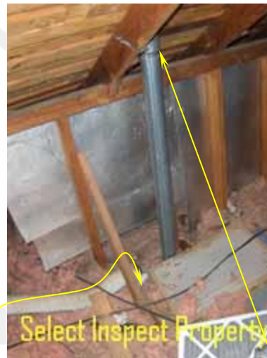
↑ other end of flex duct & water heater flue did not meet clearance requirements to combustibles
