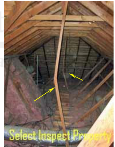
↑ failed framing
