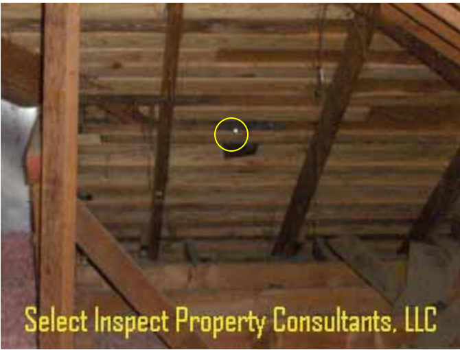
↑ daylight seen from north attic; deficient flashing suspected
