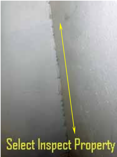
↑ example compression at hall closet
