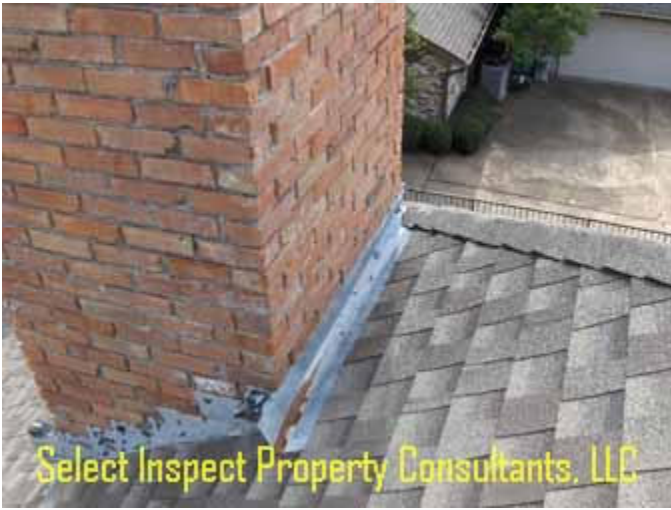
↑ Saddle/cricket should be present for water shedding at the chimney; low side flashing was lifted; moisture intrusion evidence discovered in attic
