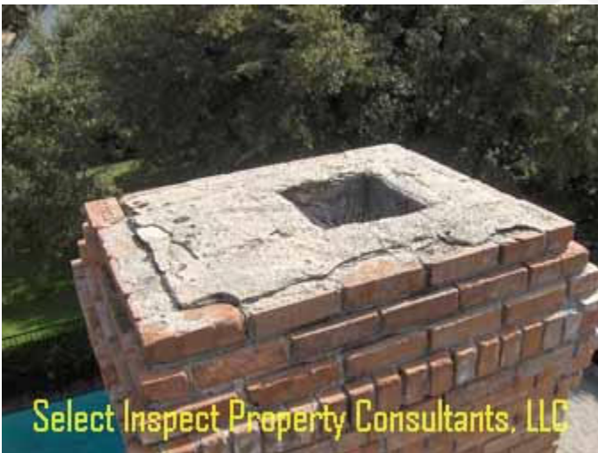
↑ chimney cap needs mortar repair & screen was inadequate
