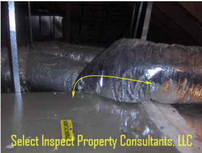
↑ crimped air ducting; example at north unit
