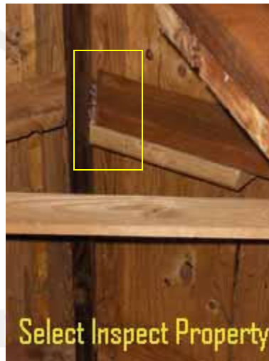
↑ rafter separation & added bracing; example at ridge
