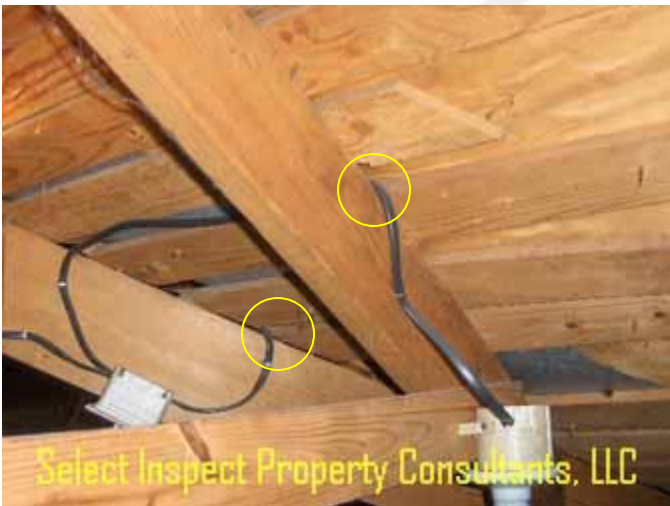
↑ wires shall not be routed between rafters & decking; example at north attic
