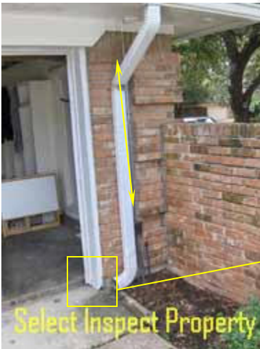
↑ inadequately secured electrical conduit & rot
