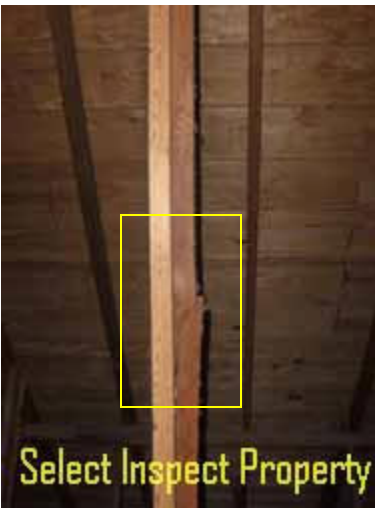
↑ failed framing
