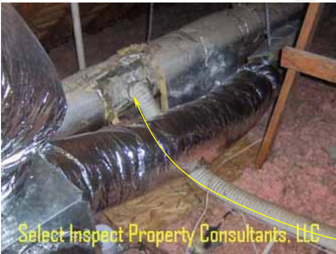
↑ unusual flex duct routed from supply to water heater closet
