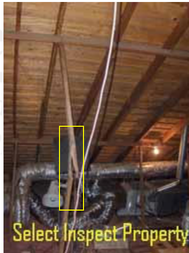
↑ failed framing
