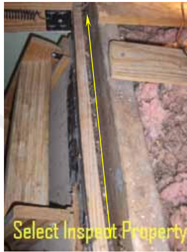
↑ missing shims at attic stair
