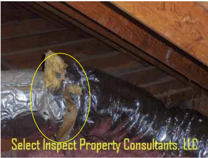
↑ deficient vapor barrier & insulation at ducting connection; example; inadequate support also noted in various locations
