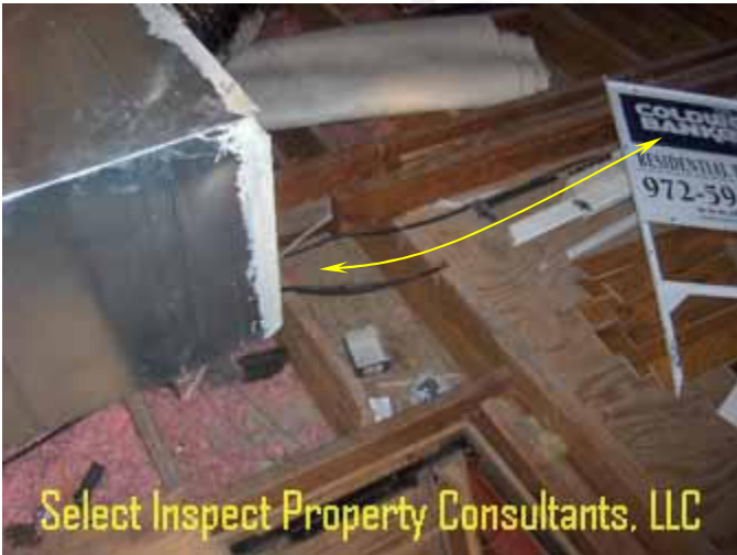
↑ electrical wires in the attic shall be adequately protected within 7' of attic stairs & electrical wires/cables shall not be routed along walking surfaces or in any location prone to traffic damage
