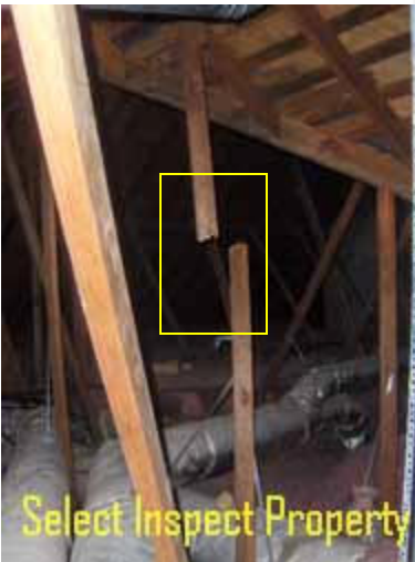
↑ failed framing
