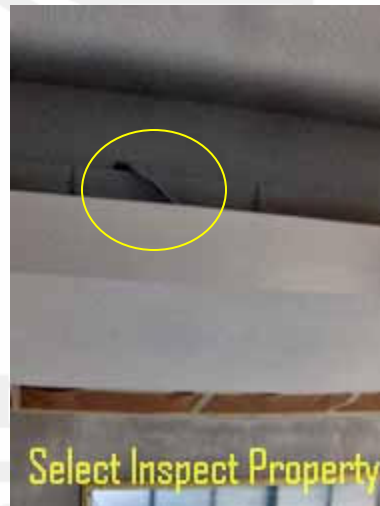
↑ questionable electrical wire routing at southeast bedroom fur down; have this checked with other electrical repairs
