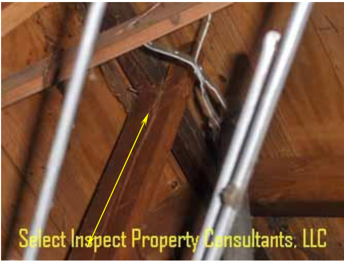
↑ cracked framing
