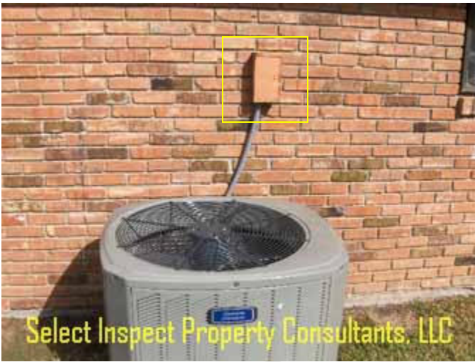
↑ incorrect location of air conditioning condenser(s) service disconnect; inadequate clearance of electrical panel for service personnel & service boxes are not to be painted
