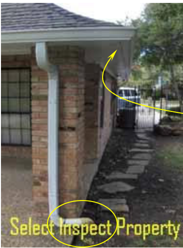
↑ deficient area drain connection & rot
