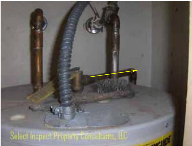
↑ water heater temperature/pressure relief drain improperly routed uphill
