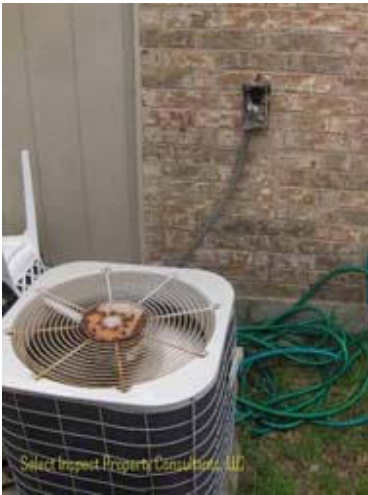
↑ incorrect location of air conditioning condenser(s) service disconnect; inadequate clearance of electrical panel for service personnel
