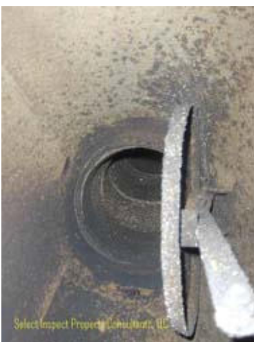
↑ fireplace interior & chimney flue need professional cleaning
