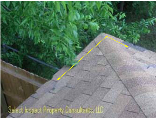
↑ tree damaged shingles at the northeast
