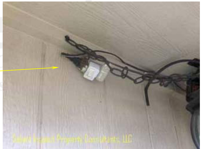
↑ close view of image at left non-exterior adaptor plugs & extension cords
