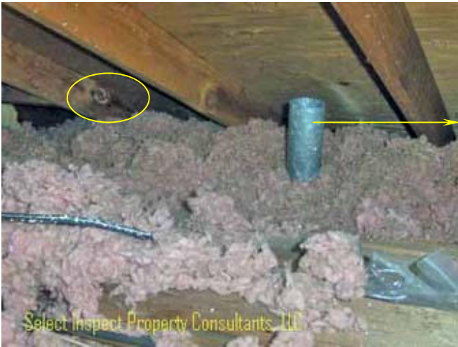
↑ knot/crack & exhaust fans improperly terminate in the attic, rather than exterior
