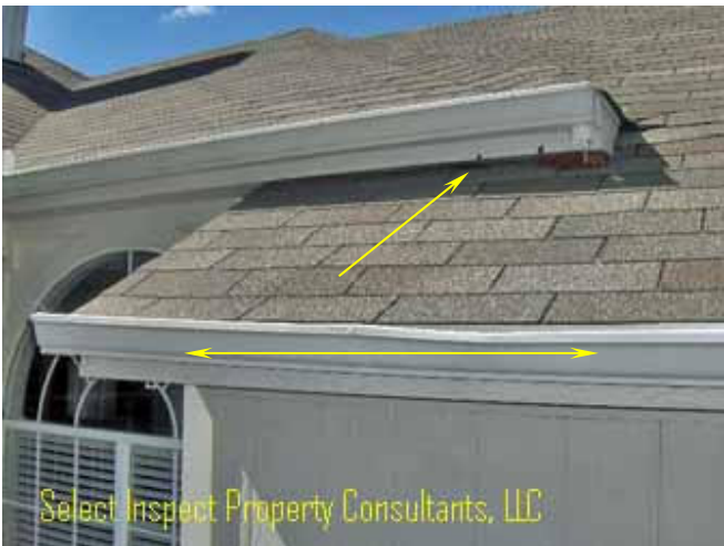
↑ moisture damage & fungus under eave & damaged guttering
