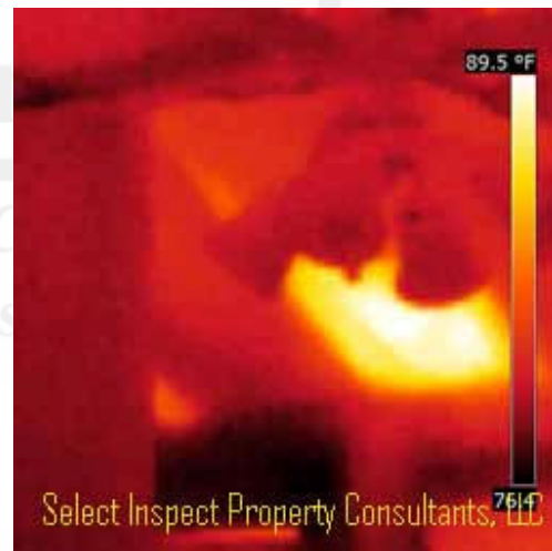
↑ Thermal imaging from square above right
