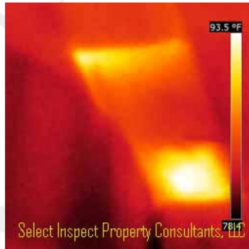
↑ Thermal imaging from square at left
