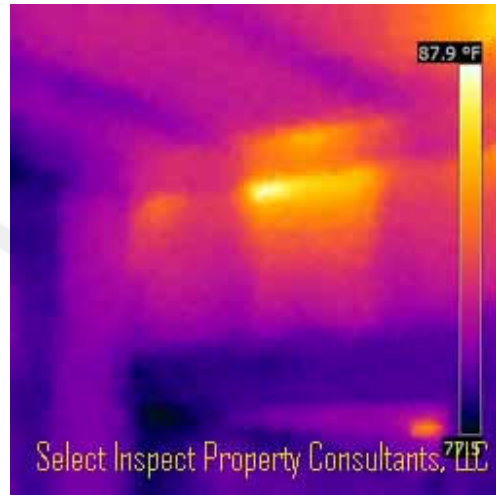
↑ Thermal imaging from square at left
