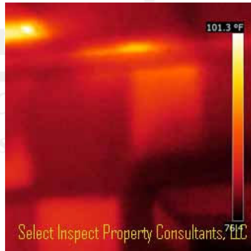
↑ Thermal imaging from square at left
