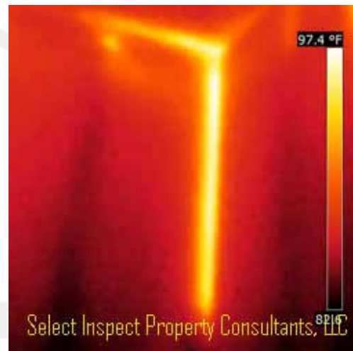
↑ Thermal imaging from square at left
