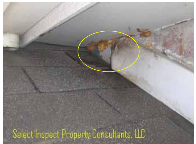
↑ short flashing, rodent damage under eave –front left
