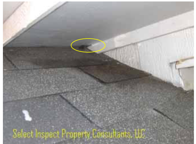
↑ missing shingles; opening, & low siding under eave; rear porch left
