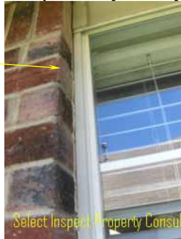
↑ close view of image at left; window separation
