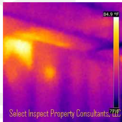
↑ Thermal imaging from square at left
