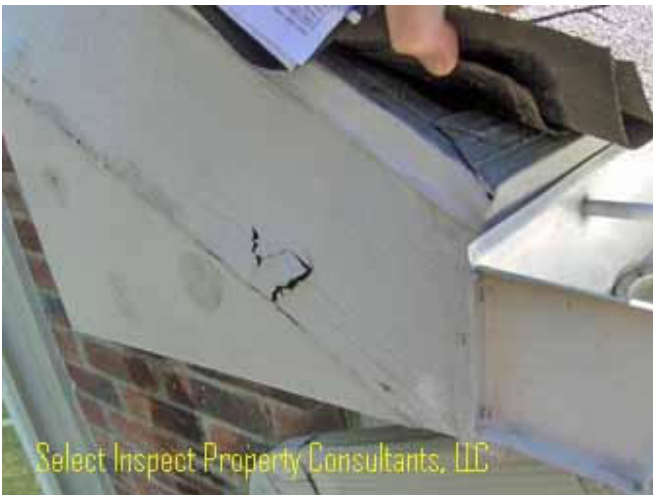
↑ moisture damage & fungus & example-unworkmanlike drip edge/felt; corners should have no gaps; rake (diagonal) edge & roof felt should be atop the eave (lower) edge flashing; roof underlayment should be under rake flashing; master northeast
