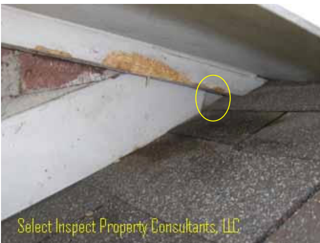
↑ short flashing, shingles, & rodent damage under eave; front right
