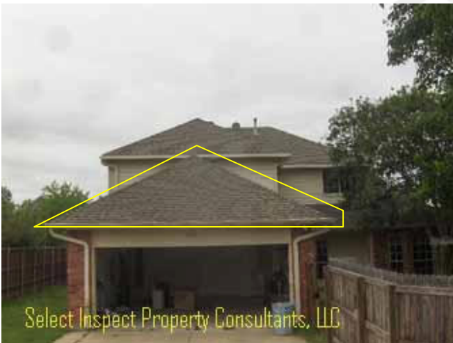
↑ missing access to this attic space; Conditions in not readily accessible/inaccessible locations remain undetermined; ie. Water heater flue, moisture stain source, electrical, framing, etc
