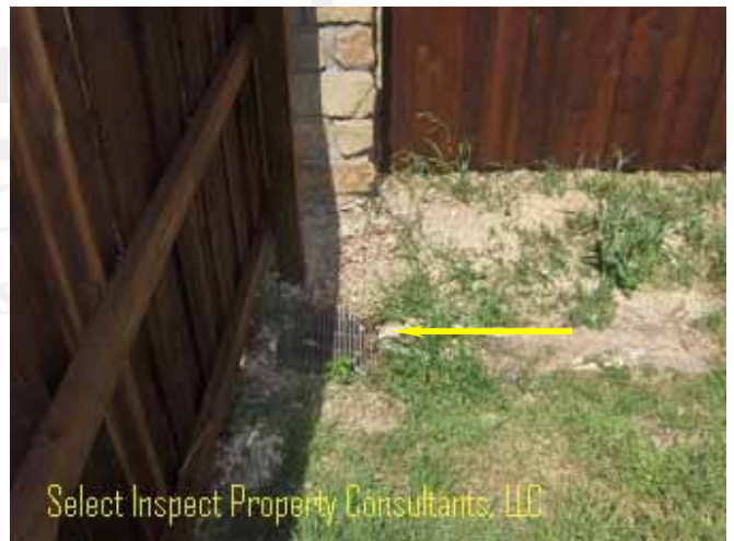
↑ an area drain termination was discovered at the far north corner
