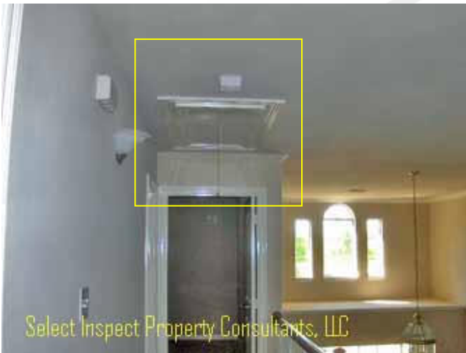
↑ energy loss at attic stair
