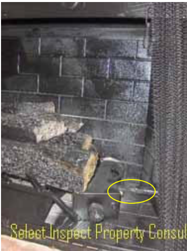
↑ disconnected fireplace logs-gas tested operable; logs not inspected
