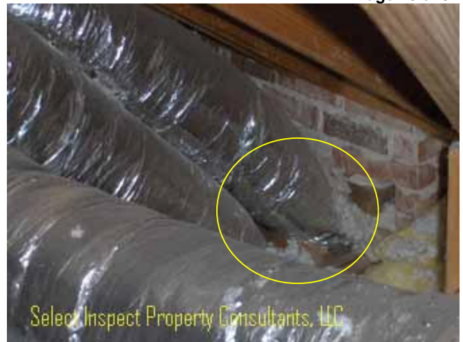
↑ crimped air ducting; example
