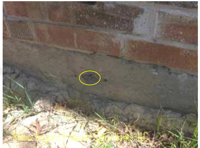
↑ exposed post tension end; example at the northwest
