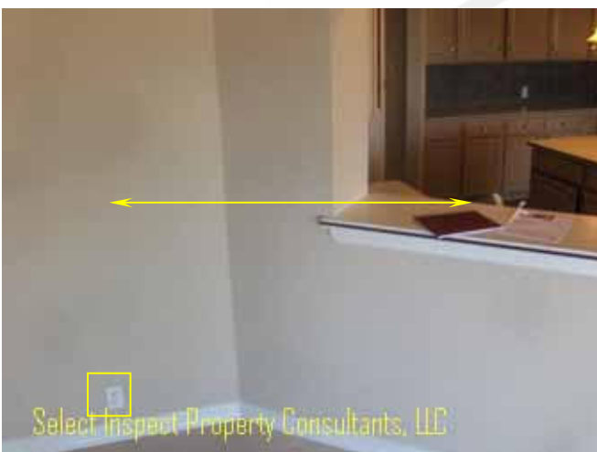
↑ GFCI required for receptacles within 6 feet of sinks; family room
