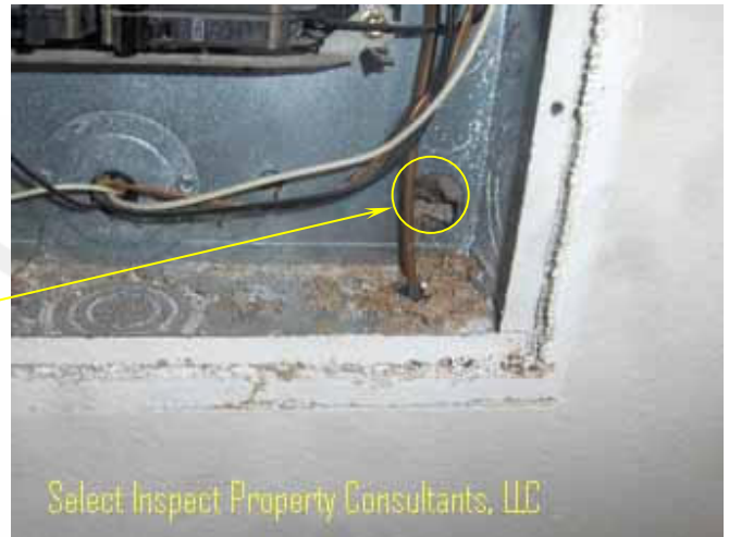
↑ close view of image at left; missing bushing at knock-out
