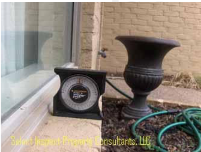
↑ brick ledge(s) had inadequate slope; example 1° rather than minimum 15°
