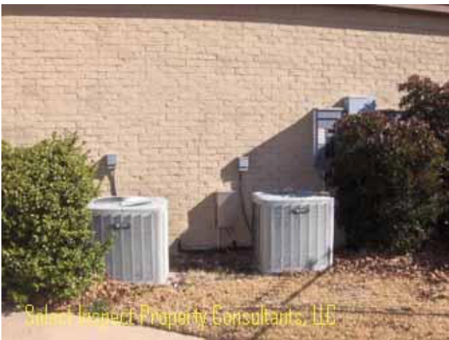
↑ incorrect location of air conditioning condenser(s) service disconnect; inadequate clearance of electrical panel for service personnel & Condensers were too low to grade- should be minimum 4" above soil
