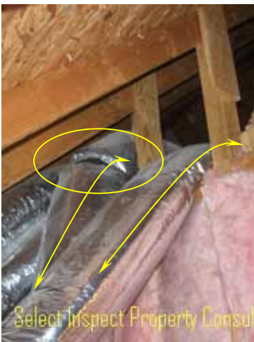
↑ walk-in attic southwest- crimped air ducting; example & deficient vapor barrier/insulation due to improper support
