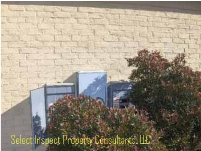
↑ Electrical service equipment requires minimum 36" clearance for access
