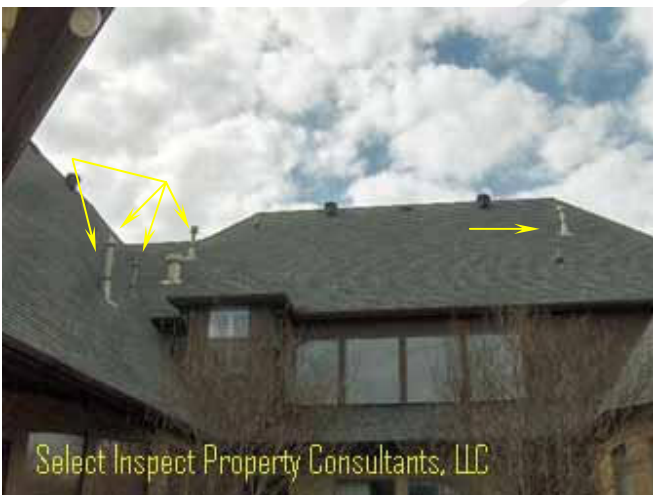
↑ flues & chimneys shall terminate at least 3 feet above the roof, and at least 2 feet above anything within 10 feet for appropriate drafting ability; *formal living area fireplace flue was not discovered in the attic or at the exterior-roof
