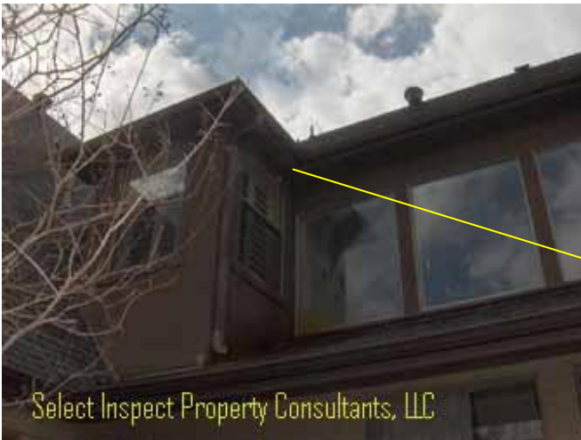
↑ auxiliary condensate drain appeared to have retracted into the eave; potential moisture damage condition
