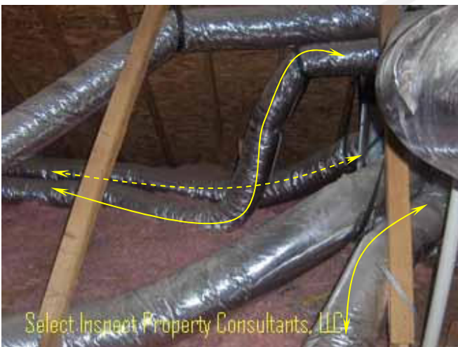
↑ inadequate support of air ducting; example location of multiple deficiencies discovered in all attic areas
