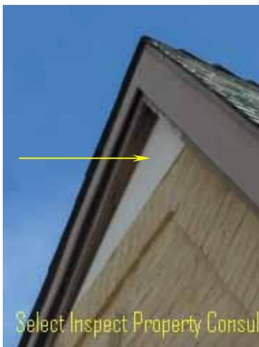
↑ northwest gable insert was inadequately secured; openings exist
