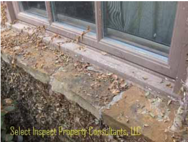
↑ example deficient mortar & sealant at windows; stone mortar is unconventional method/deep-set. This & excess ivy conditions are prone to premature wear & moisture intrusion
