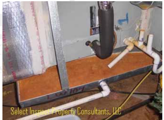
↑ same as left; other upper attic unit
