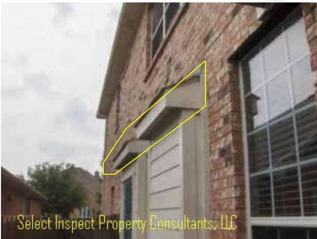
↑ unvented enclosed attic spaces; master bathroom
