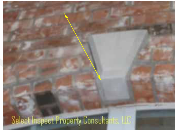
↑ stress cracks
