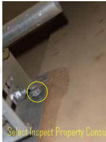
↑ inadequate fastening of overhead door spring assembly
