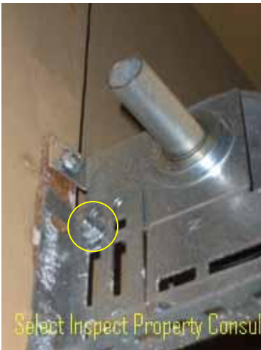
↑ inadequate fastening of overhead door spring assembly
