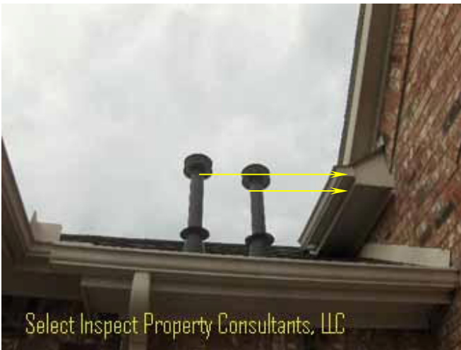
↑ water heater flues too short/close to wall
