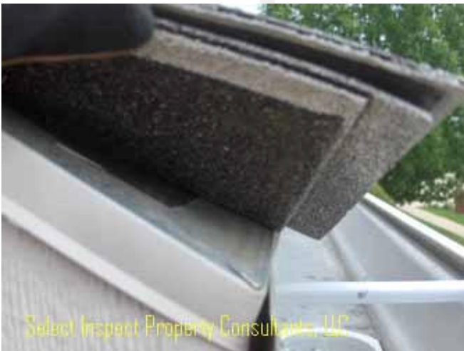
↑ example-unworkmanlike drip edge/felt; corners should have no gaps; rake (diagonal) edge & roof felt should be atop the eave (lower) edge flashing; roof underlayment should be under rake flashing
