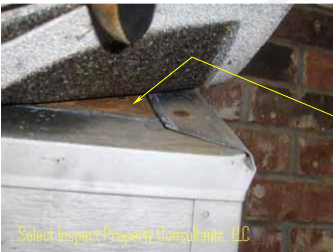
↑ missing roof underlayment at gable “eyebrow(s)” & master bathroom small roofs; example
