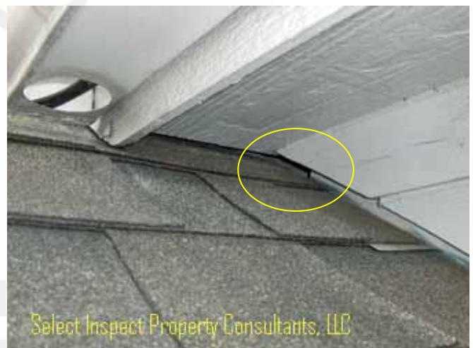
↑ opening; deficient flashing- example
