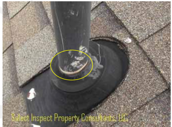
↑ vent separation & openings; example
