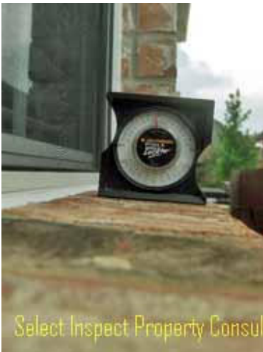
↑ brick ledge(s) had inadequate slope; example
