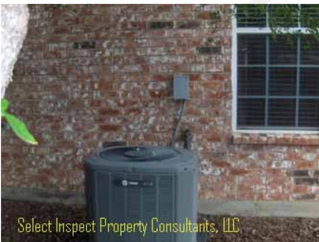
↑ example (1 of 3 discovered) incorrect location of air conditioning condenser(s) service disconnect; inadequate clearance of electrical panel for service personnel
