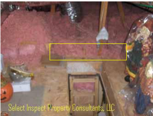
↑ there should be a minimum 24" pathway to the HVAC from the top of the access, with no gaps or obstructions
