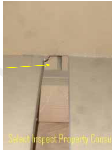
↑ close view of image at left opening at garage drywall between levels; visible framing
