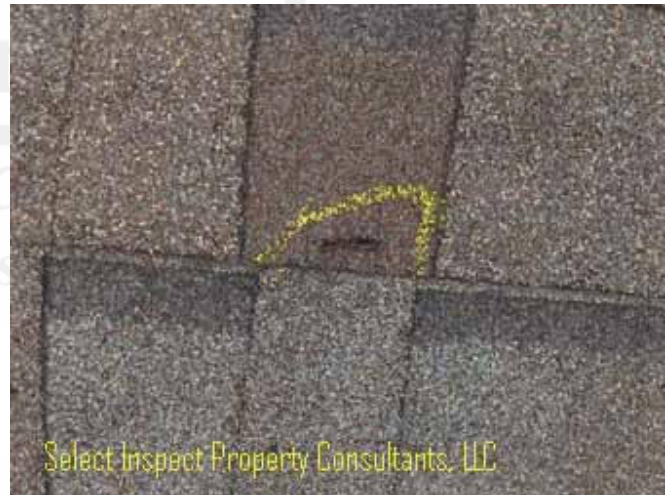
↑ popped/exposed roof staple; example
