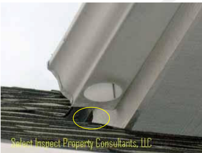
↑ opening; damaged fascia- upper left of front porch
