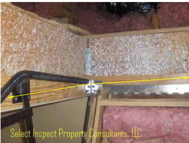
↑ improper/inadequate fasteners at attic stair; unworkmanlike & unsafe
