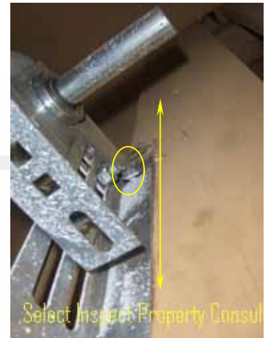
↑ inadequate fastening of overhead door spring assembly & cracked framing
