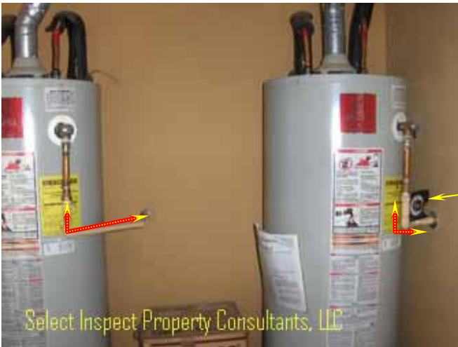
↑ cpvc sections of water heater temperature/pressure relief piping was smaller than required by the device manufacturer
