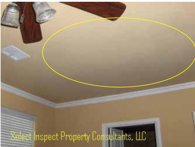
↑ repair evidence at master bedroom
