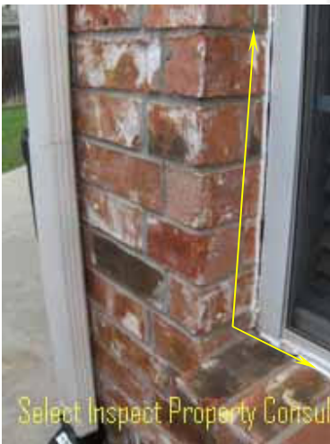
↑ window separation; stress
