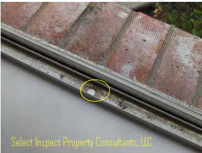
↑ Alarm holes at the lower portion of the window may allow moisture intrusion; caulk and monitor
