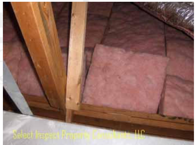
↑ unworkmanlike insulation
