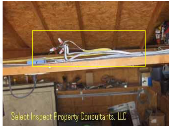
↑ unworkmanlike/unsafe wiring- example at east garage
