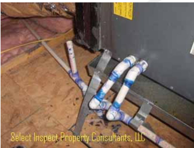
↑ unworkmanlike combining of primary condensate drain & auxiliary condensate drain drains; & air conditioning primary condensate drain should be insulated
