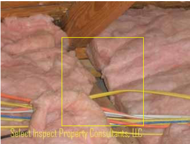
↑ unworkmanlike insulation
