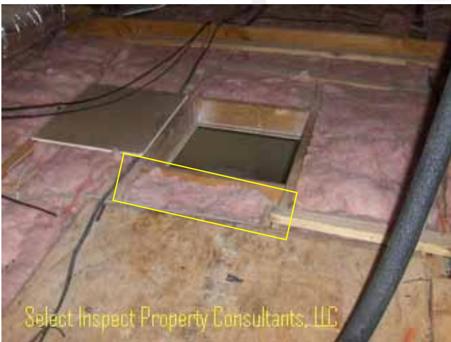
↑ there should be a minimum 24" pathway to the HVAC from the top of the access, with no gaps or obstructions; attic hatch was also too small for removal/service of mechanical equipment
