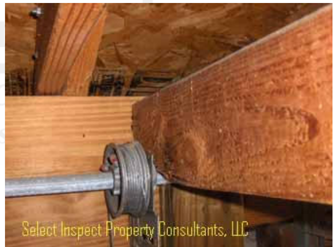
↑ undersized joist; inadequate connection; unworkmanlike notching; example of multiple similar conditions
