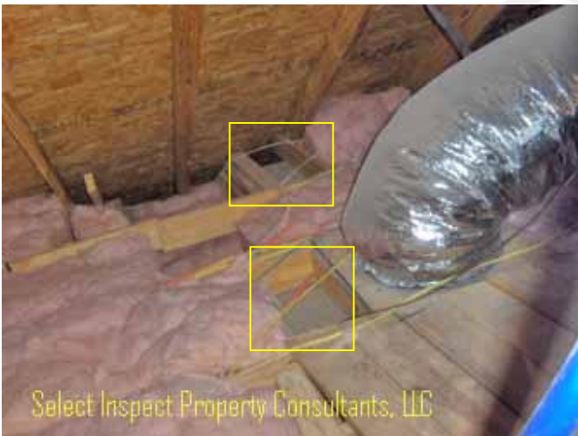
↑ unworkmanlike; missing insulation
