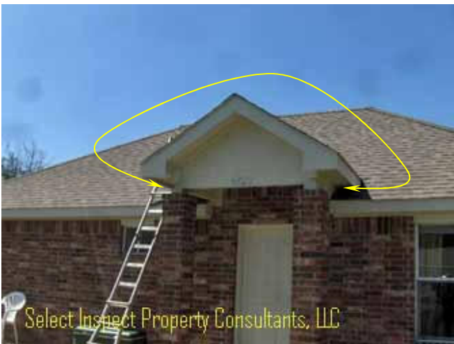
↑ missing flashing; openings; visible roof deck & attic components & example of wood too close to roofline
