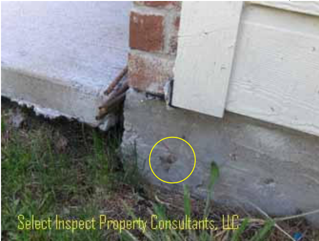
↑ exposed post tension end(s) at the west
