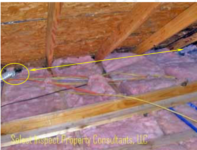
↑ unworkmanlike insulation; obstructing eave/soffit vents; also in this picture: exhaust fan(s) improperly terminate in the eaves, rather than to the exterior
