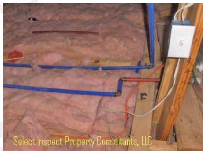
↑ unworkmanlike insulation
