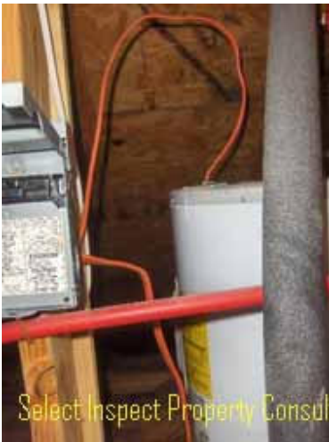
↑ Wires should be secured within 12 inches of junction boxes, switches, receptacles, fixtures
