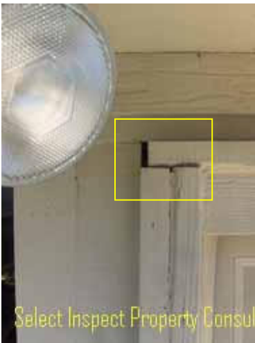
↑ holes at siding, trim, overhead doors, wall air conditioning etc. should be sealed; example at left overhead door
