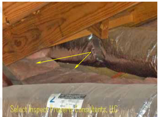
↑ unworkmanlike insulation
