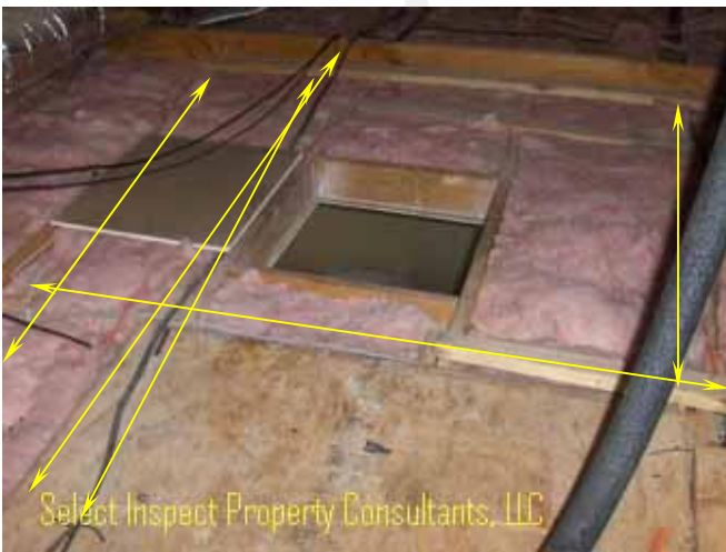
↑ electrical wires in the attic shall be adequately protected within 6' of attic scuttle or within 7' of attic stairs; & electrical wires/cables shall not be routed along walking surfaces or in any location prone to traffic damage
