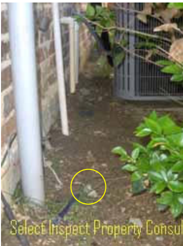
↑ grounding electrode protrudes grade; deficient
