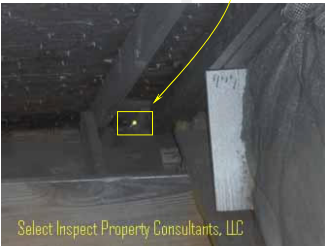
↑ attic location of above images; daylight seen from inside
