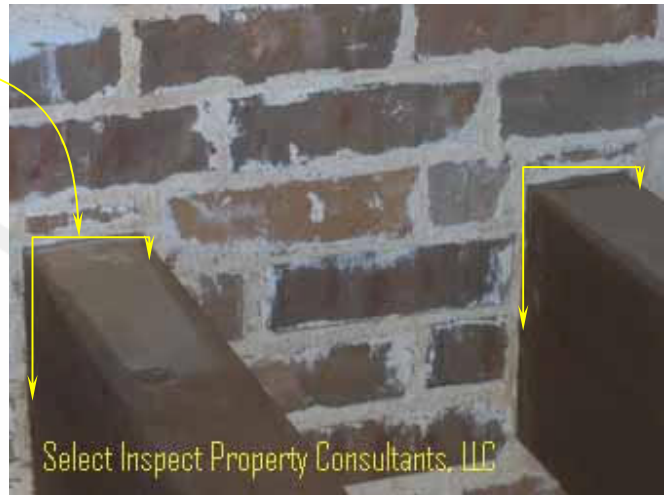
↑ sealant recommended at beam joints at brick
