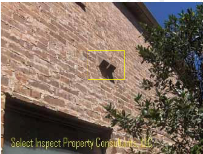
↑ some exhaust fans appeared to terminate at the exterior- correct
