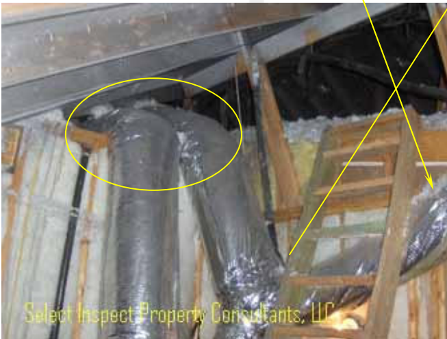
↑ crimped air ducting; example
