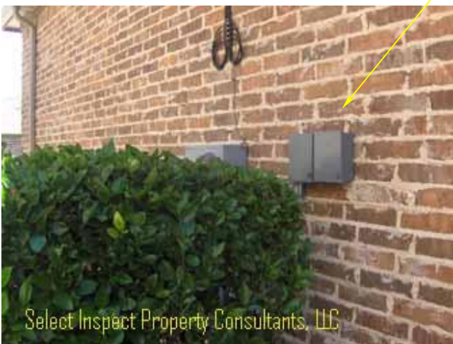
↑ inadequate clearance at air conditioning condenser(s) service disconnects
