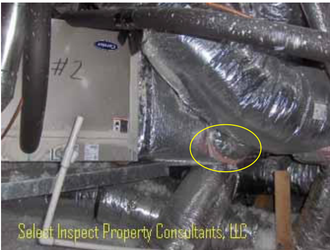
↑ inadequately sealed duct to plenum; corrosion (likely from condensation) & energy loss
