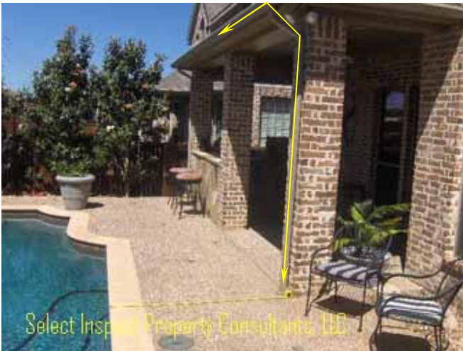
↑ metal gutter near pool; refer to an electrician for bonding options
