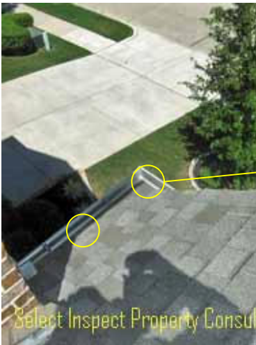
↑ protruding nail; split shingle
