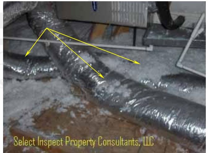
↑ crushed ducting below HVAC
