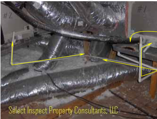
↑ air conditioning primary condensate drain should be insulated; traps not discovered
