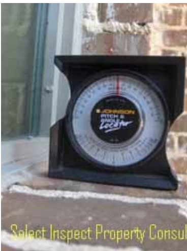
↑ brick ledge(s) had inadequate slope; example at front- 1 °
