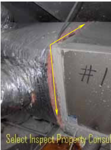
↑ inadequate seal at plenum/component joints & energy loss discovered; example
