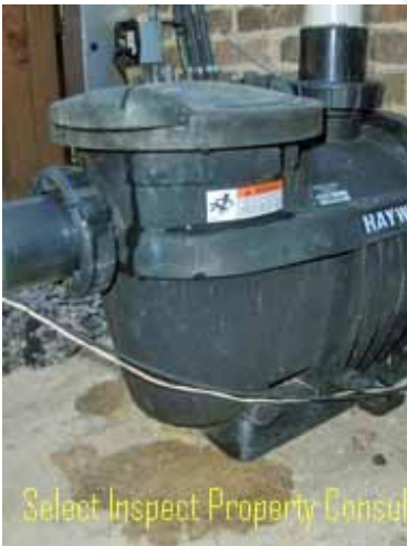
↑ leakage discovered at pool pump
