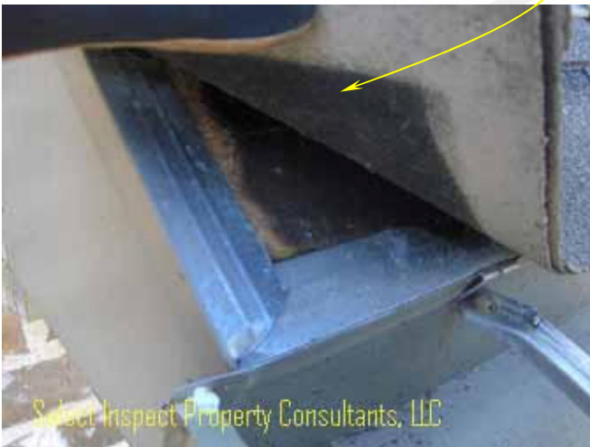
↑ short cut roof underlayment corners should have no gaps & rake (diagonal) edge & roof felt should be atop the eave (lower) edge flashing & under rake flashing
