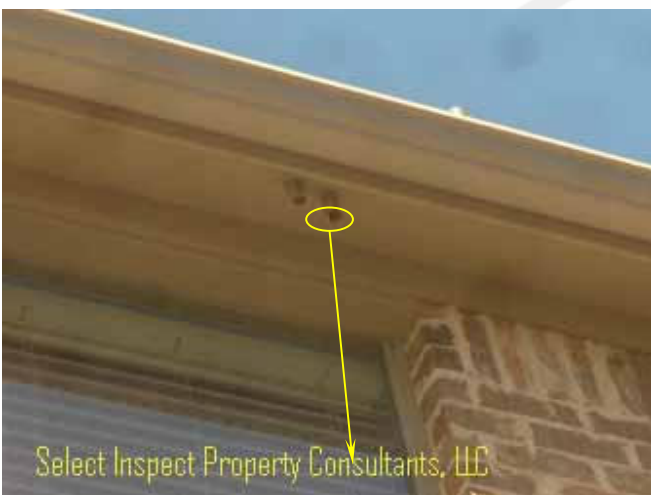
↑ stains indicate history of auxiliary condensate drainage
