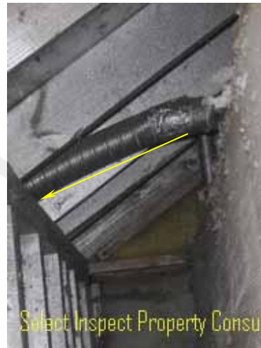
↑ exhaust fan(s) improperly terminate in the eaves, rather than to the exterior
