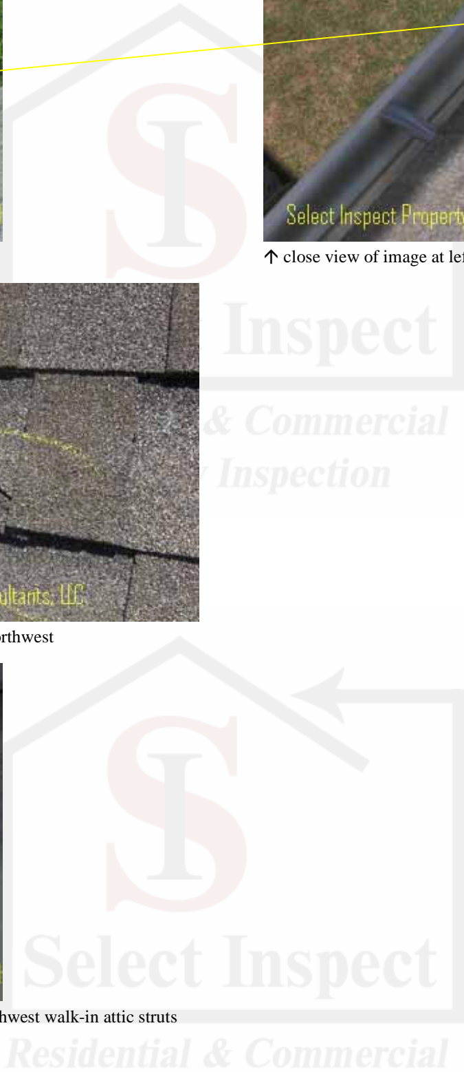
↑ protruding nail; split shingle
