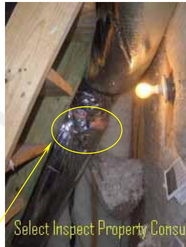
↑ deficient ducting & inadequate support of air ducting; example
