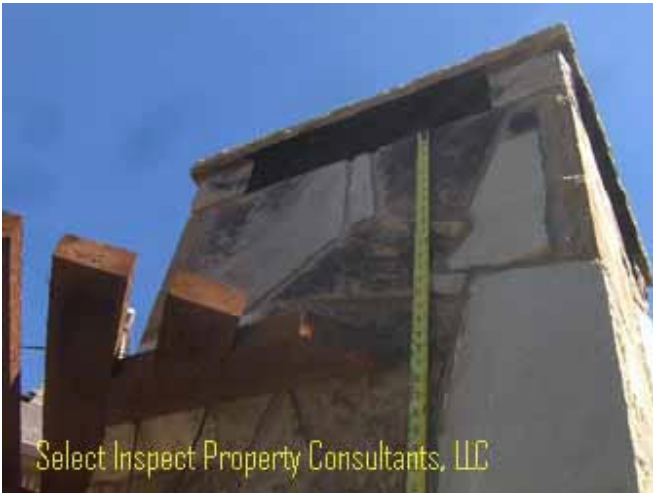
↑ Arbor was less than 2' below chimney termination; flues & chimneys shall terminate at least 3 feet above the roof, and at least 2 feet above anything within 10 feet
