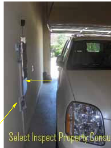
↑ inadequate clearance at electrical cabinet; cover not removed, interior not inspected
