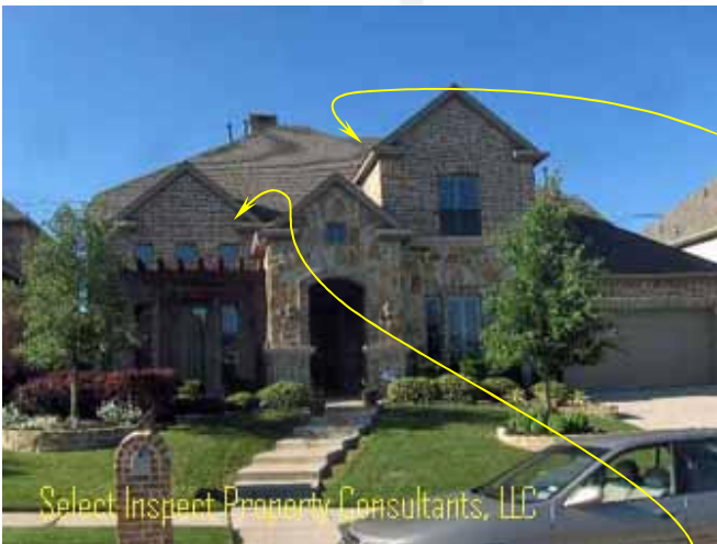
↑ unworkmanlike deck -unworkmanlike drip edge/felt;
