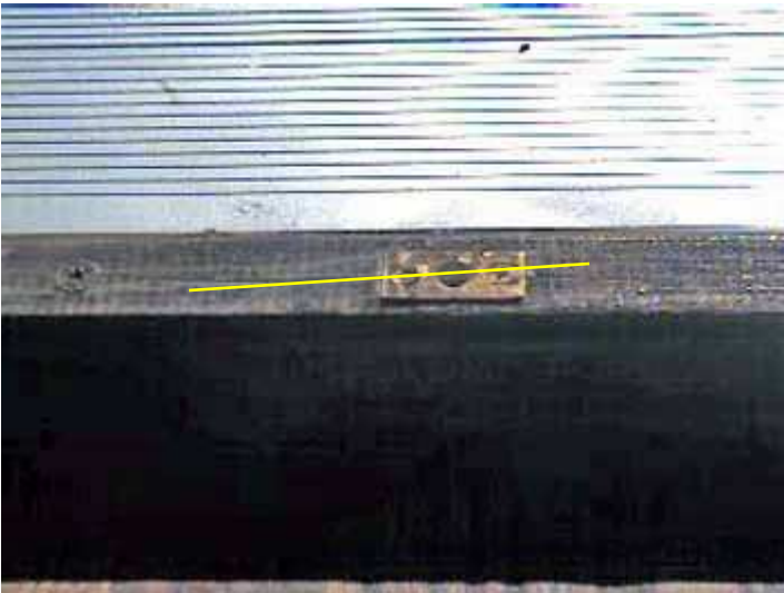
↑ cracked threshold at front entry doorway
