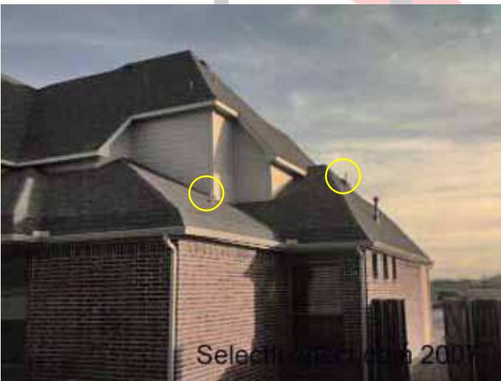
↑ capped plumbing vents at west-northwest
