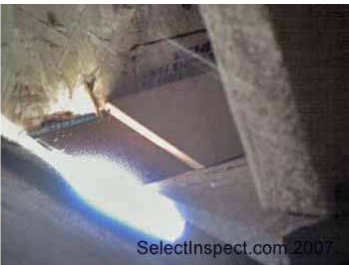
↑ close view of prior image- opening / daylight visible
