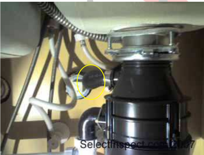
↑ crimped dishwasher drain tube
