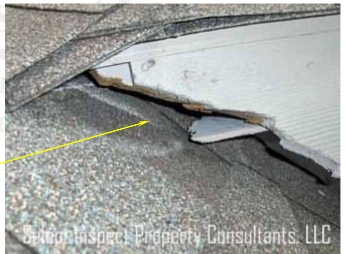
↑ close view of image at left; large enough for moisture intrusion & or rodent/bird entry
