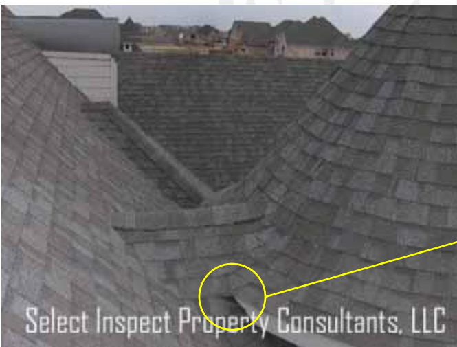
↑ opening remains at rotunda fascia; attic framing visible from exterior
