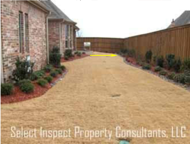
↑ satisfactory slope at west-southwest
