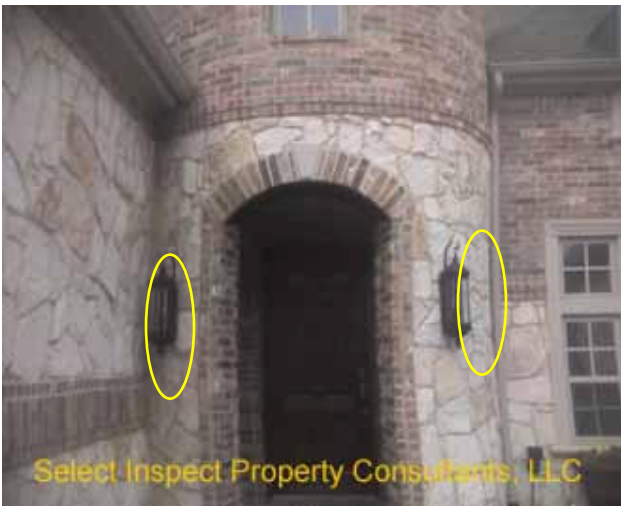
↑ seal top of exterior lights; example front entry
