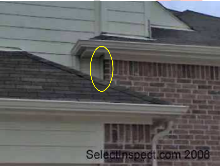
↑ openings and converging valley example at right garage
