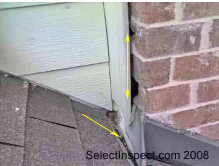
↑ close view of prior image- openings and low slope at small valley- upper right garage
