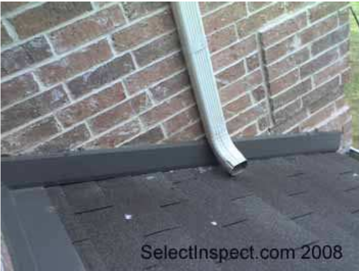
↑ correct counter flashing at opposite side of front porch roof
