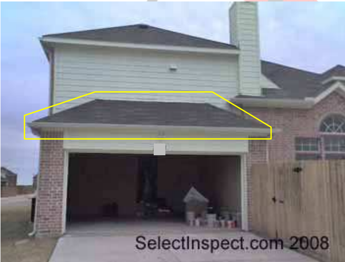
↑ unvented garage attic
