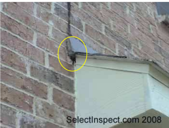
↑ close view of prior image- moisture and pest intrusion concern
