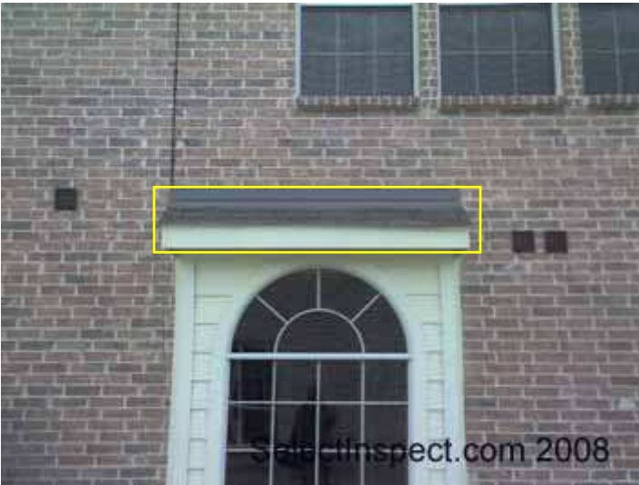
↑ unvented enclosed attic at master bathroom window
