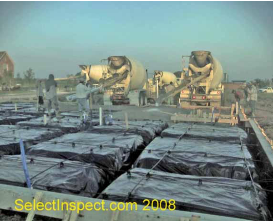
↑ the master bedroom, bathroom, & closet areas were poured first
