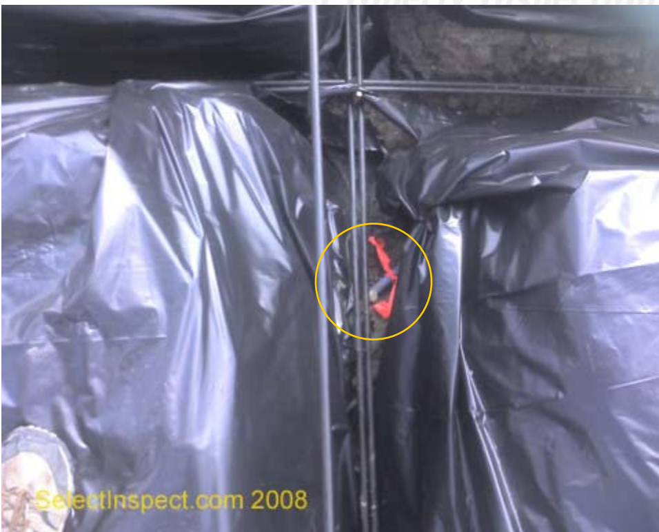
↑ close view of image above
