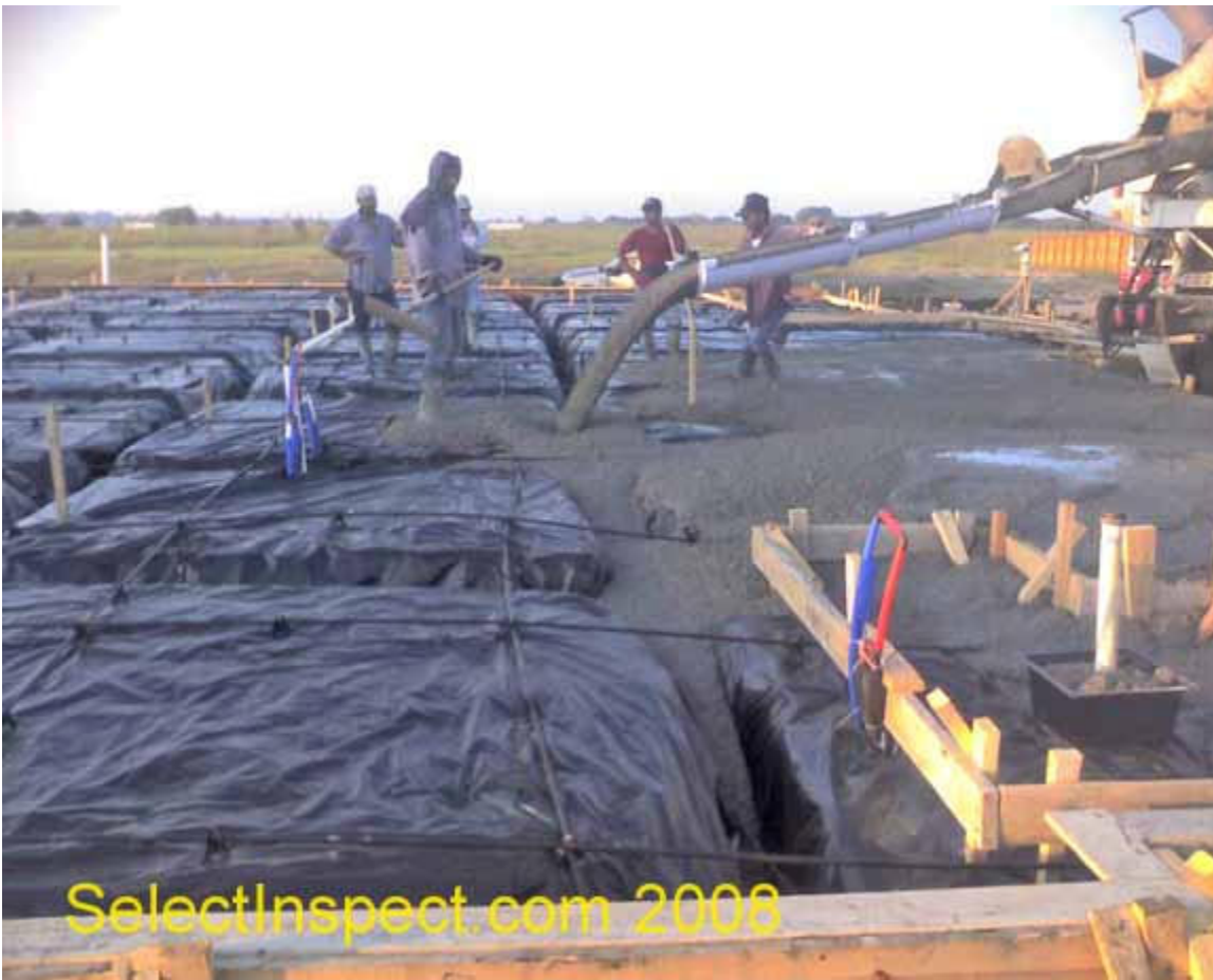
↑ trenches are filled, then the pads
