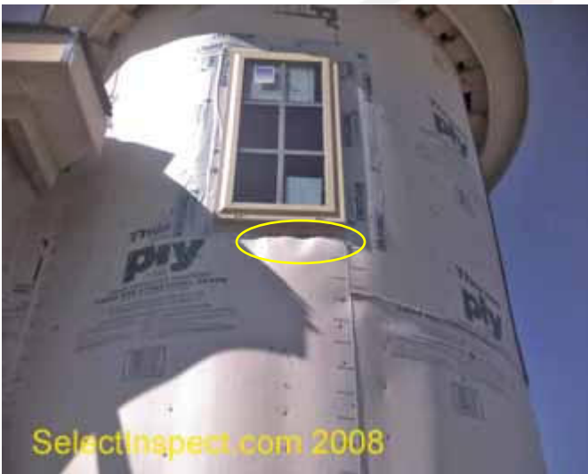
↑ marginal flashing at window
