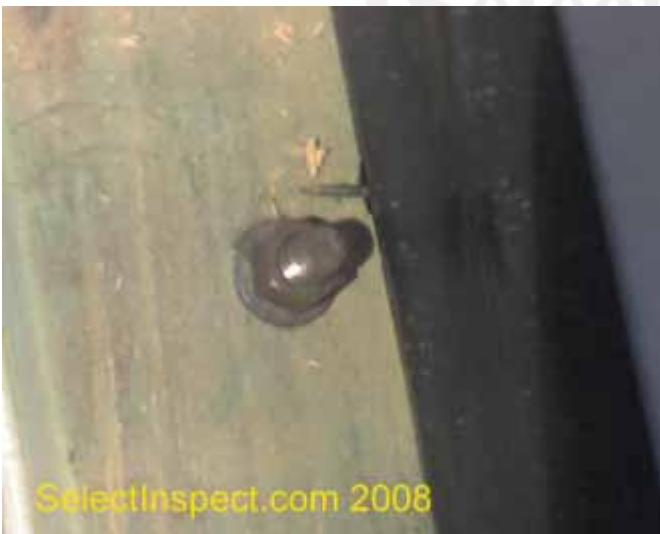
↑ appropriate anchor installation; example
