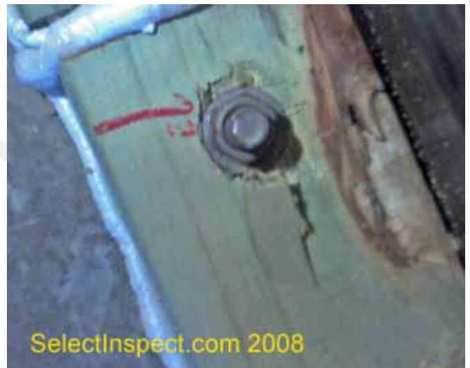
↑ over tightened anchor; example
