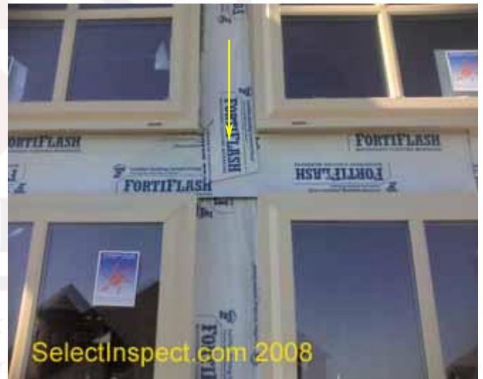
↑ correct lapping of flashing; example
