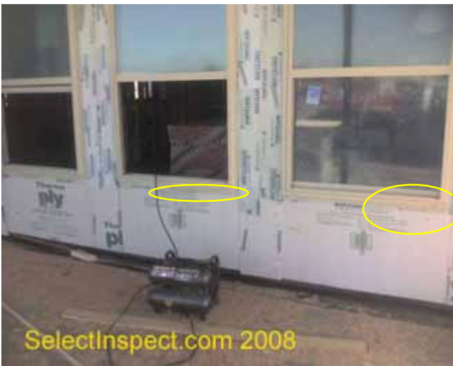
↑ marginal flashing at windows
