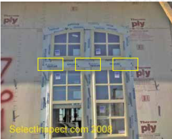
↑ improper lapping of window flashing; example
