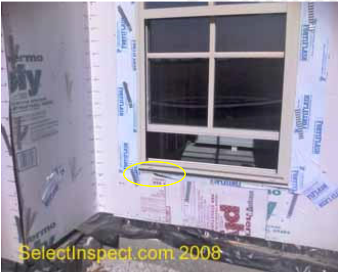
↑ marginal flashing at bedroom 2 south window
