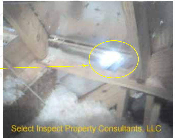
↑ attic view of image at left; opening & daylight visible
