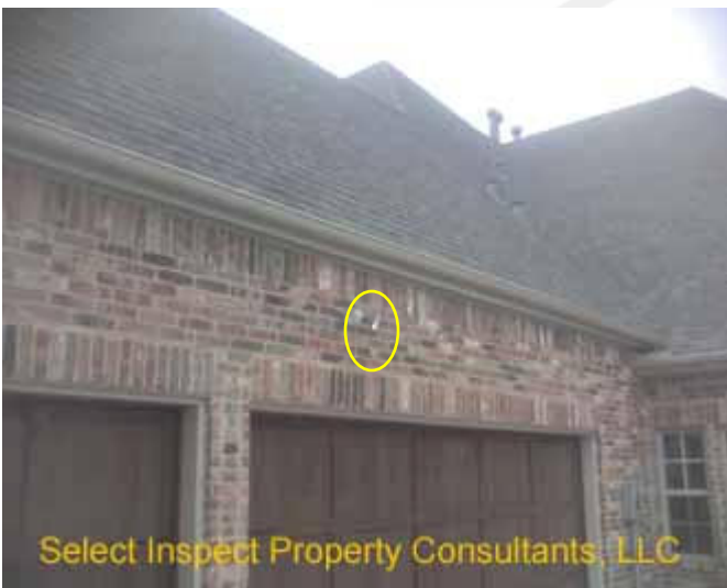
↑ seal top of exterior lights; garage
