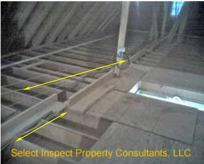
↑ Unprotected electrical wires within 6 feet of scuttle or 7 feet of attic stair
