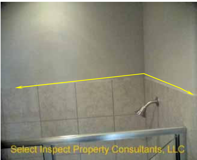
↑ Seal the top tile edge at the shower walls- example at split bathroom
