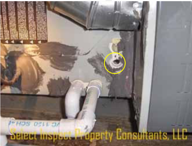
↑ missing evaporator(s) plug at the north #3 HVAC
