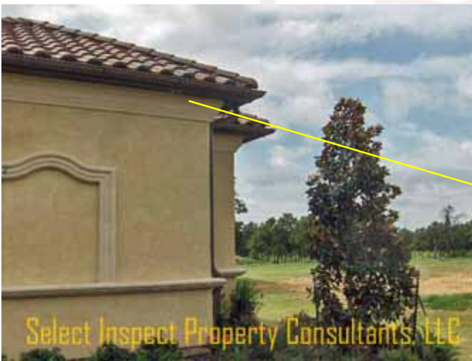
↑ slightly askew soffit vent example; Significant issues were not discovered
