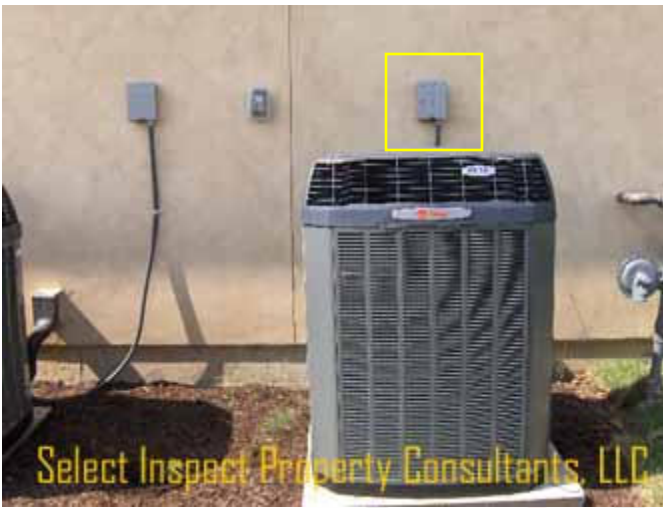
↑ incorrect location of air conditioning condenser(s) service disconnect; example
