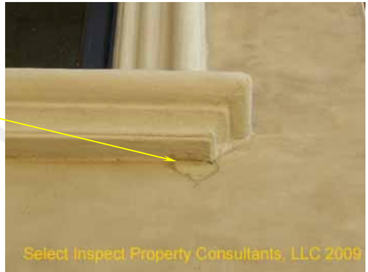
↑ close view of image at left
