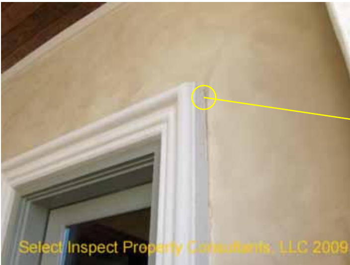
↑ opening at Artificial Stucco; driveway door
