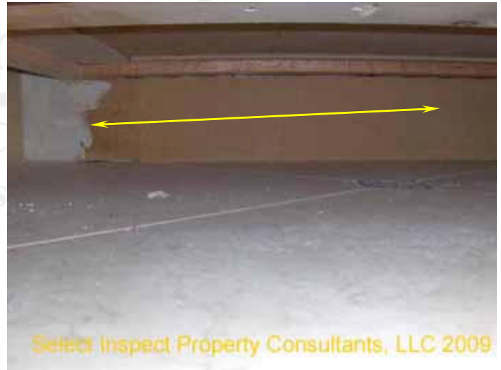
↑ same as image at left; under sink cabinet
