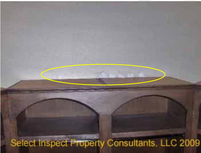
↑ incomplete paint finish; example above master closet cabinets
