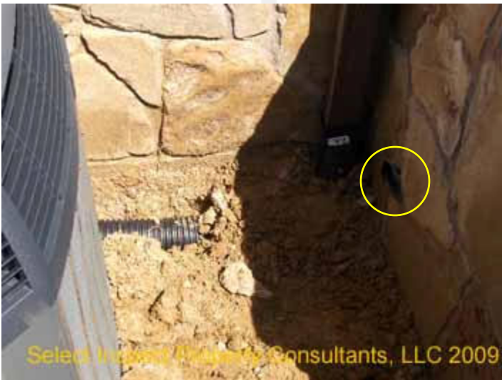
↑ improper termination of area drain at the southeast
