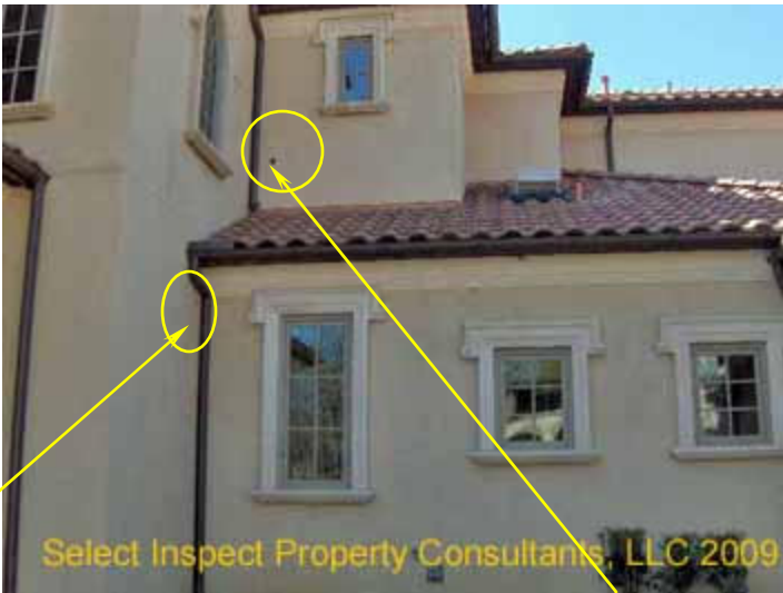
↑ openings at eastern walls near garage
