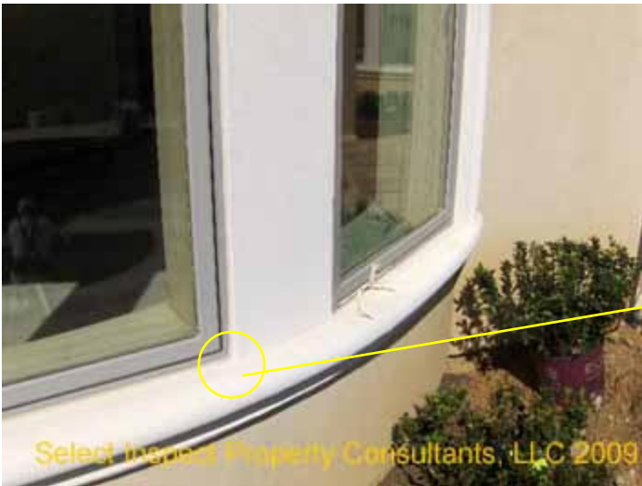
↑ cracked veneer at the master bedroom sill
