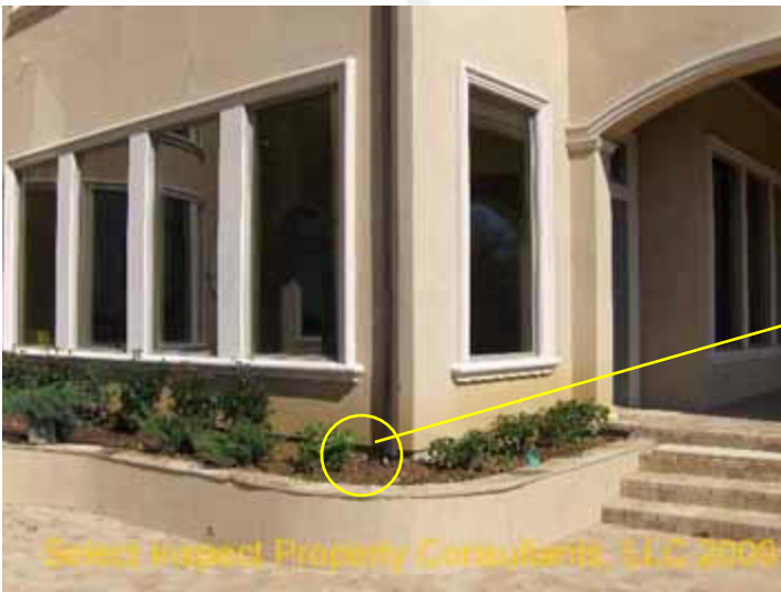
↑ exposed conduit at slab adjacent the family room
