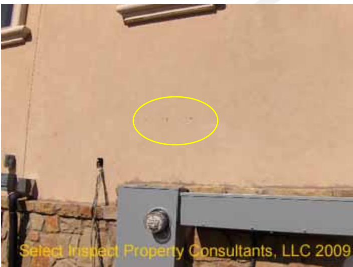
↑ openings above the electrical service
