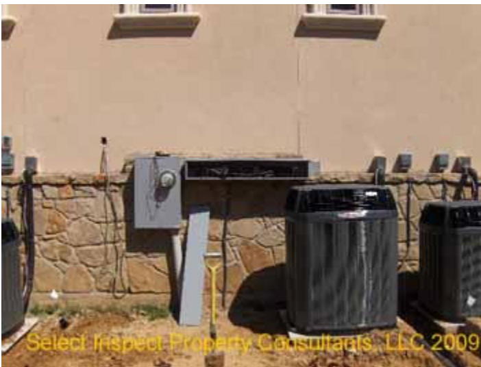
↑ improperly located air-conditioner electrical disconnect(s)
