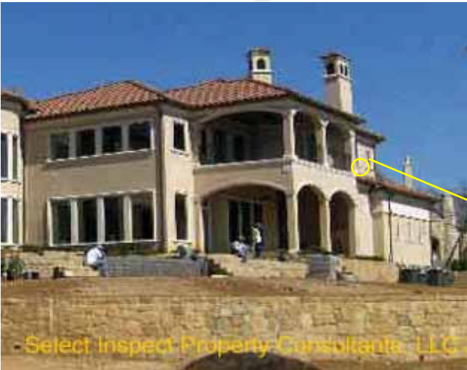
↑ opening exists at flashing
