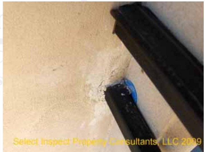
↑ additional example of railing at stucco wall
