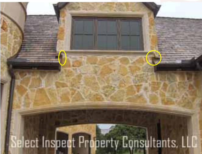
↑ sealant recommended at flashing details
