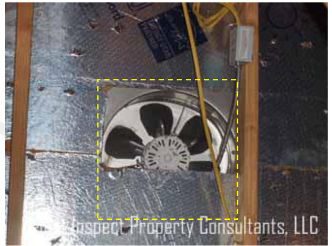
↑ small fan opening above HVAC #4; upper attic from bedroom #3
