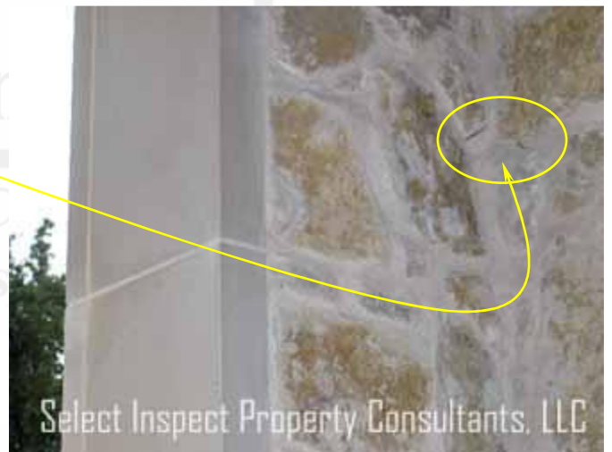
↑ nails at the front porch
