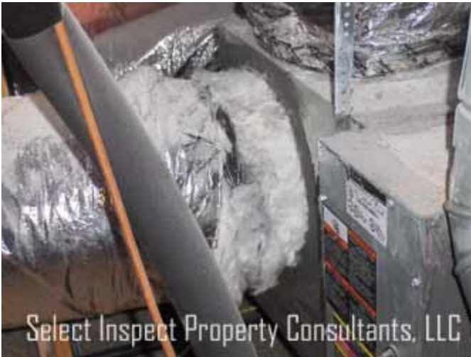
↑ deficient insulation & vapor barrier at HVAC #1; north attic
