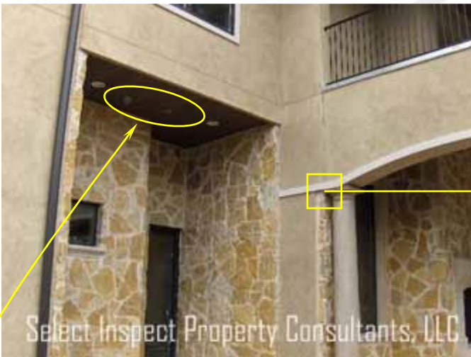
↑ deficient exhaust fan(s) termination & mortar tuck-pointing needed at north patios
