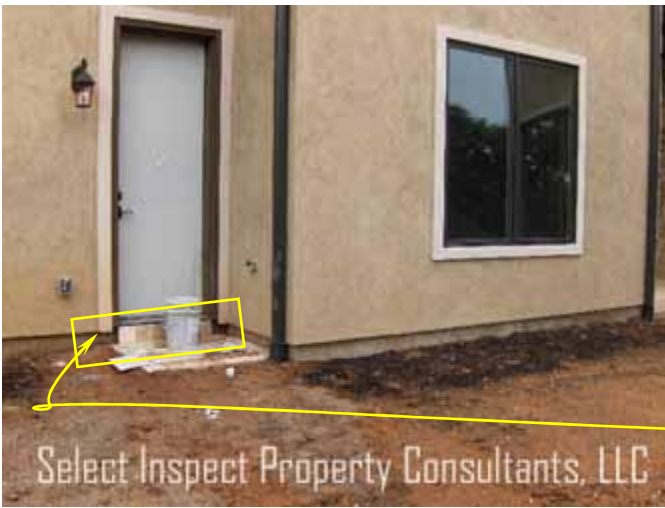
↑ recommend painting/sealing all exposed wood; example
