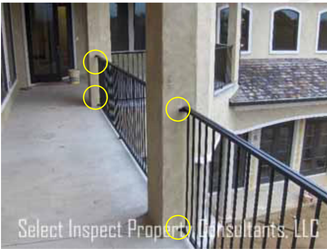
↑ railing install has scratched finish at balcony columns; example
