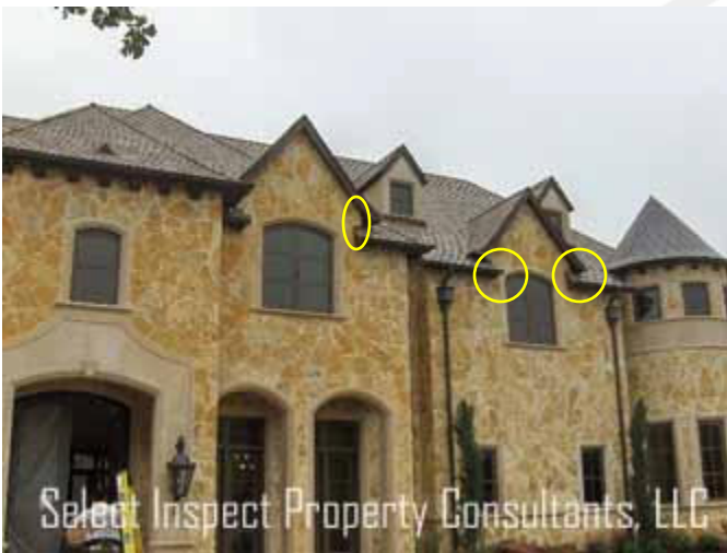
↑ same as above; seal flashing details
