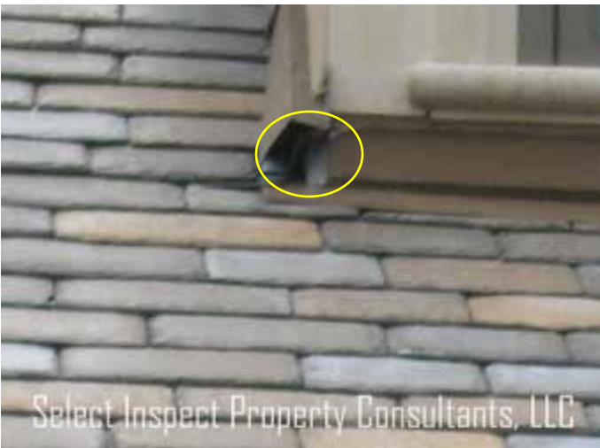
↑ opening at left dormer flashing detail
