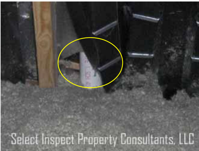
↑ no obvious deficiencies found in the attic below the image above
