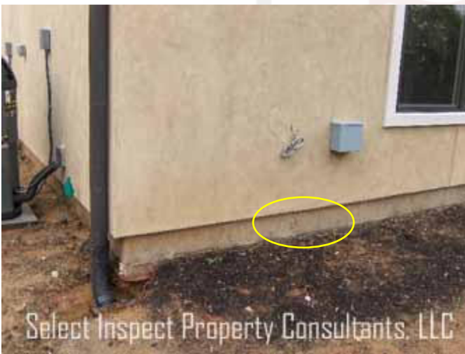
↑ exposed post tension end(s) cap at the north; three-car garage
