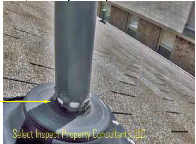
↑ close view of image at left; seal & monitor
