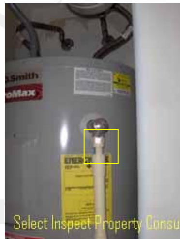
↑ temperature/pressure relief piping at this section was smaller than required by the device manufacturer
