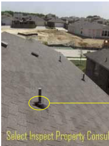
↑ plumbing vent separation implies settlement of the roof structure & or raising of the vent stack
