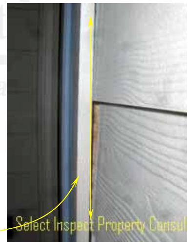
↑ close view of image at left; wall substrate/vapor barrier visible
