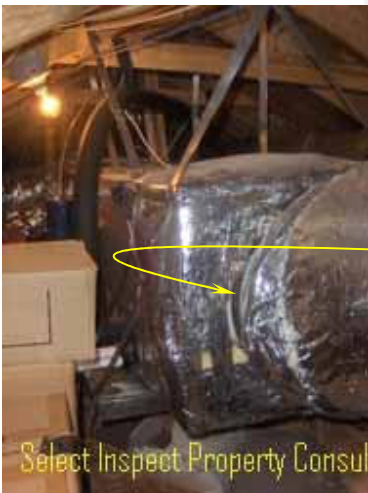
↑ return air duct remains inadequately secured & inadequately sealed
