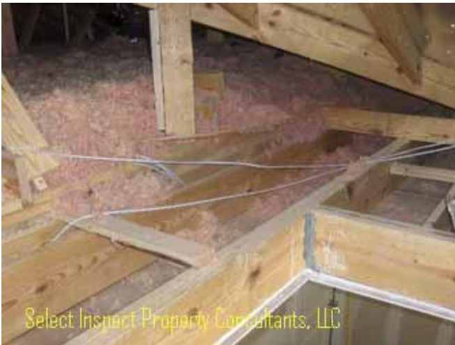
↑ electrical wires in the attic shall be adequately protected within 6' of attic scuttle; unworkmanlike electrical remains in the attic
