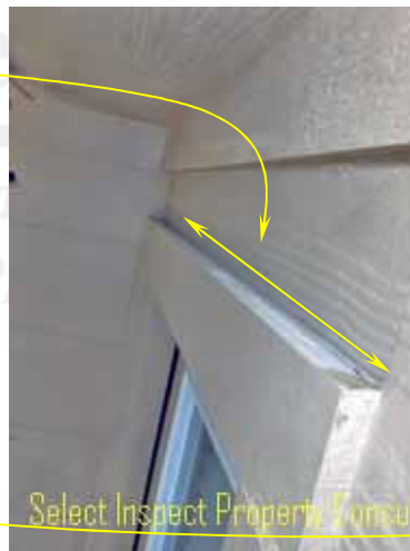
↑ close view of image at left; open at top of door trim
