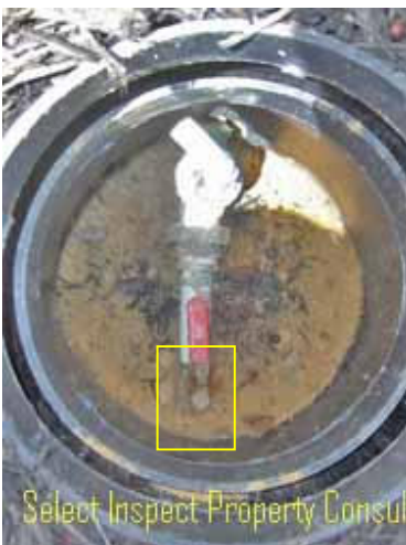
↑ rust/corrosion at auxiliary water shut-off-valve; Shut-off-valves require 3" clearance from soil
