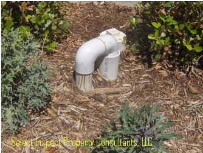
↑ "air-gap" (atmospheric pressure break) was not present / inadequate for the pool system
