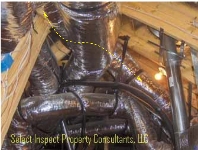
↑ crimped air ducting; example
