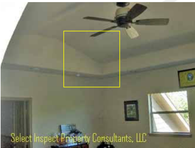
↑ Thermal imaging implies energy loss at gameroom northwest
