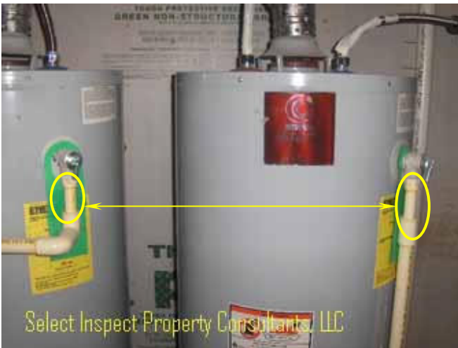
↑ temperature/pressure relief piping at these sections was smaller than required by the device manufacturer
