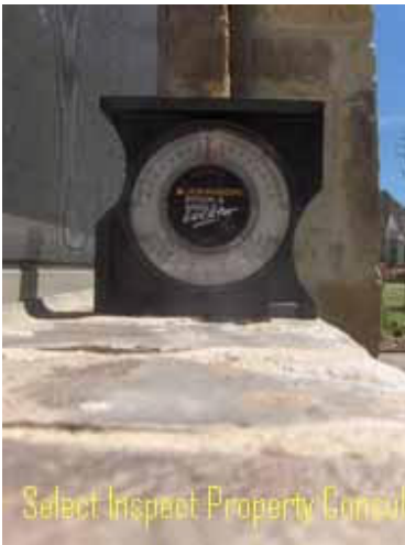
↑ brick ledge(s) had inadequate slope; example of 2 ° at front window
