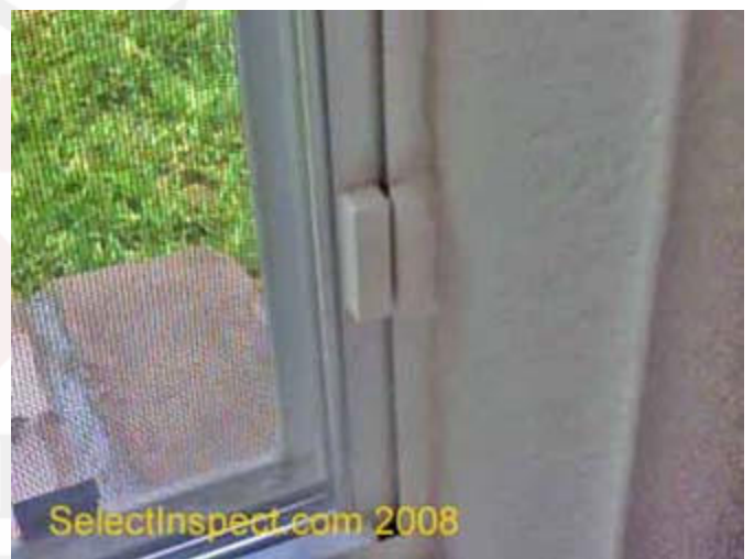
↑ Alarm holes at the lower portion of the window may void manufacturer warranty; ** recommended method
