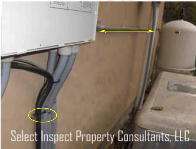
↑ sealant needed at equipment boxes/penetrations
