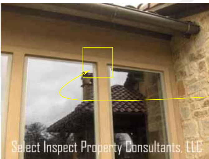
↑ unworkmanlike window corner example
