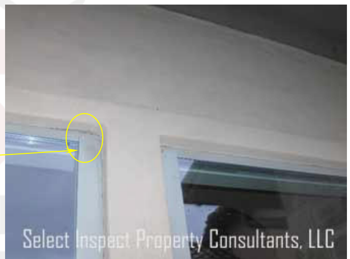
↑ close view of image at left; Significant issues were not discovered; monitor & maintain
