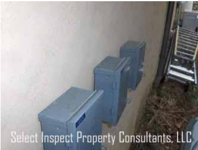
↑ sealant needed at all equipment boxes/penetrations
