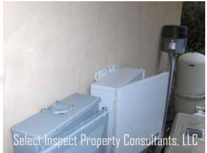
↑ sealant needed at all equipment boxes/penetrations
