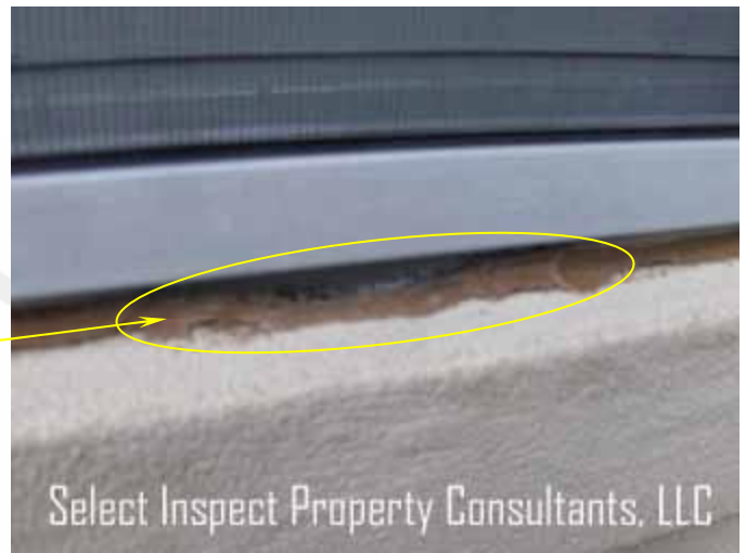
↑ close view of image at left; openings at stucco along window; example
