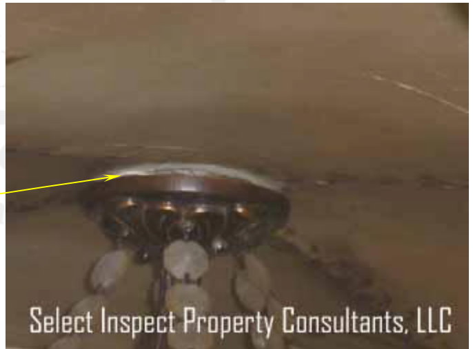
↑ close view of image at left; may be inadequately secured
