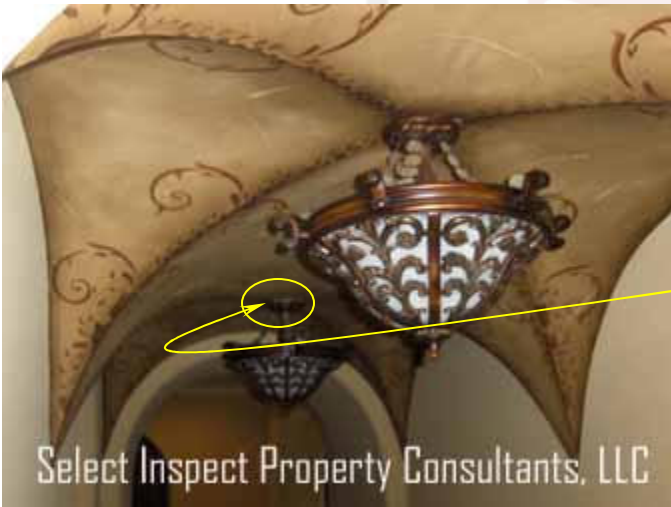
↑ excess reveal; example at gallery lights
