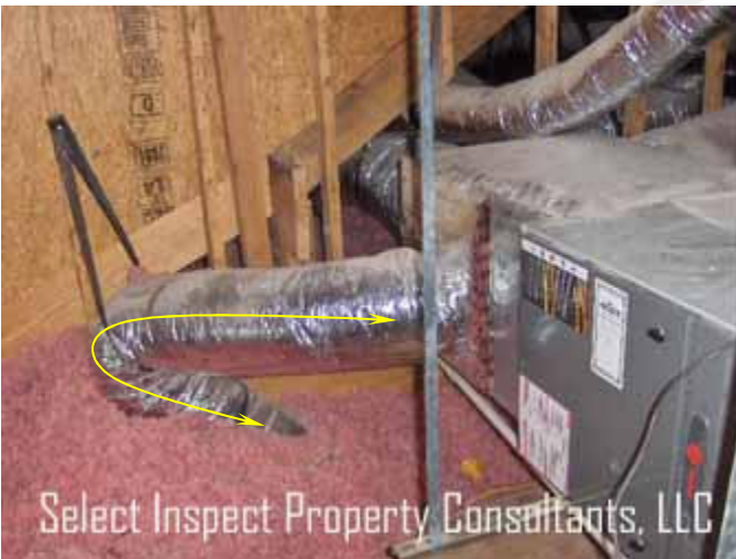
↑ crimped air ducting; example
