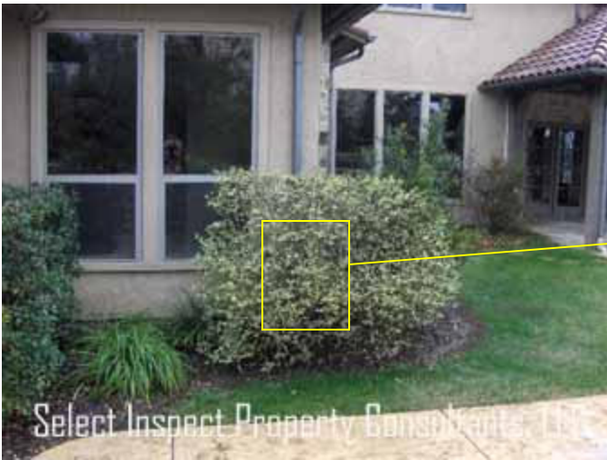
↑ sealant needed at equipment penetrations
