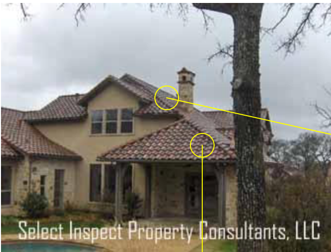
↑ deficient/cracked tiles
