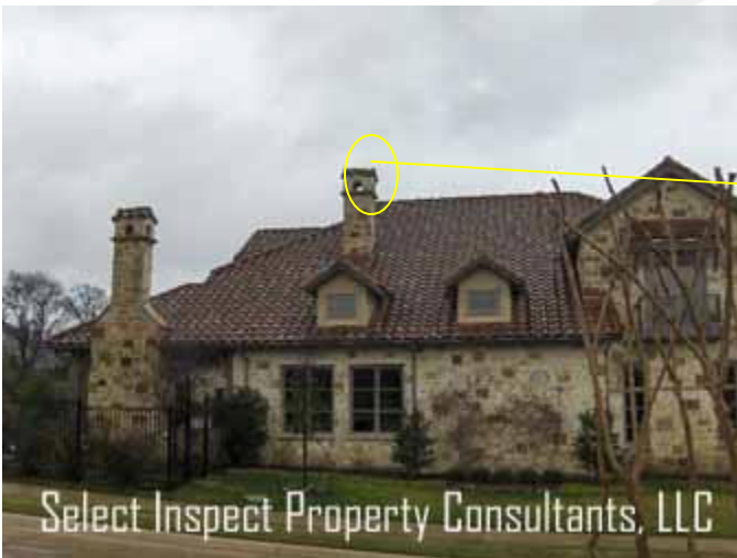
↑ missing tile at chimney; back side of chimneys & some other high or otherwise concealed roof areas were inaccessible/undetermined
