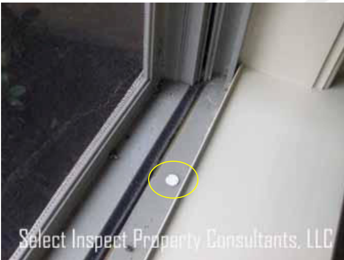
↑ Alarm holes at the lower portion of the window may void manufacturer warranty; ** recommended method
