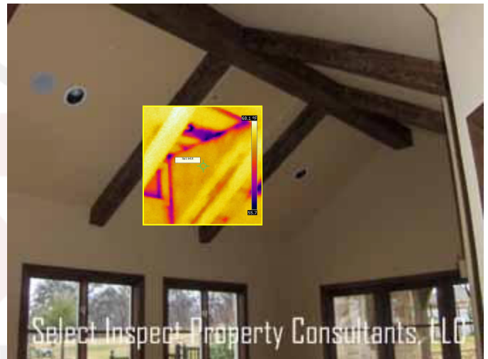
↑ darker thermal areas imply apparent lacking insulation or other "cooler" areas from suspected air infiltration discovered at vaults & recessed lights; example at breakfast nook dormer
