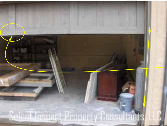
↑ sealant needed & protruding nails
