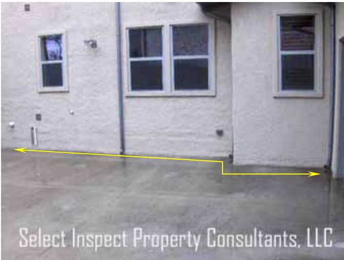
↑ stucco drainage plane/screed at/below concrete grade
