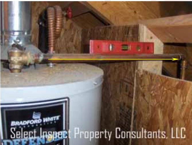
↑ two-car garage water heater; uphill (slightly) temperature/pressure relief
