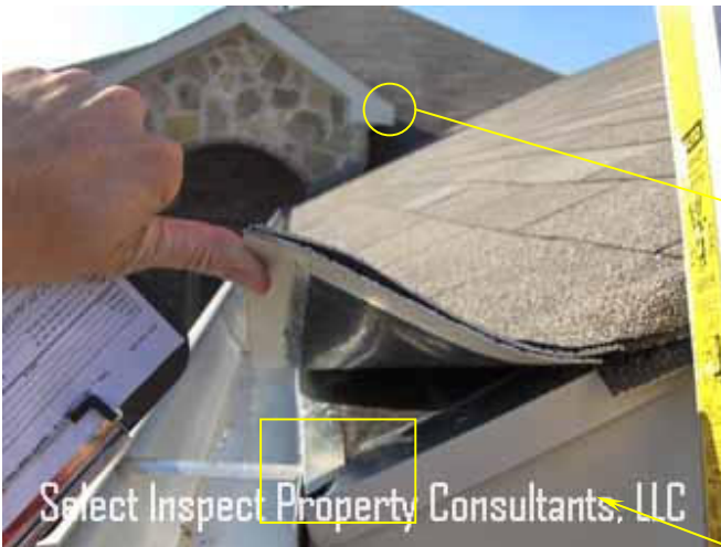
↑ unworkmanlike drip edge/felt; corners should have no gaps & rake (diagonal) edge & roof felt should be atop the eave (lower) edge flashing
