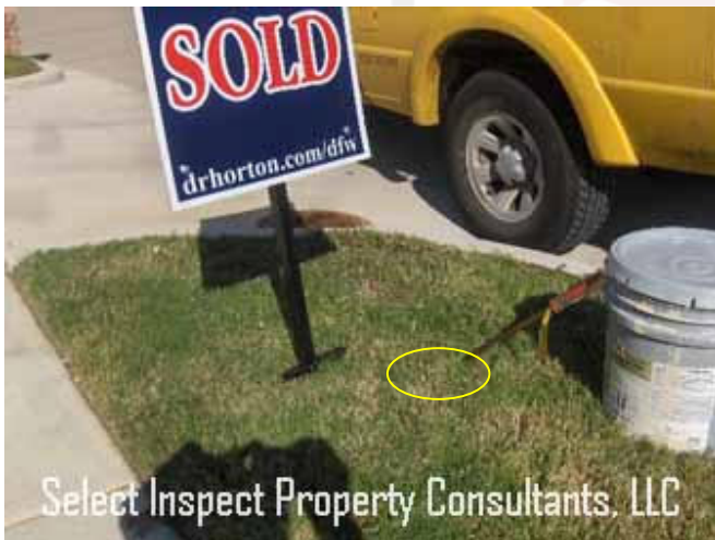
↑ irrigation tube was damaged near the driveway at this location
