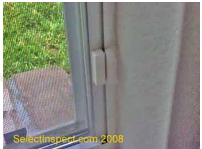
↑ Alarm holes at the lower portion of the window void manufacturer warranty; ** recommended method
