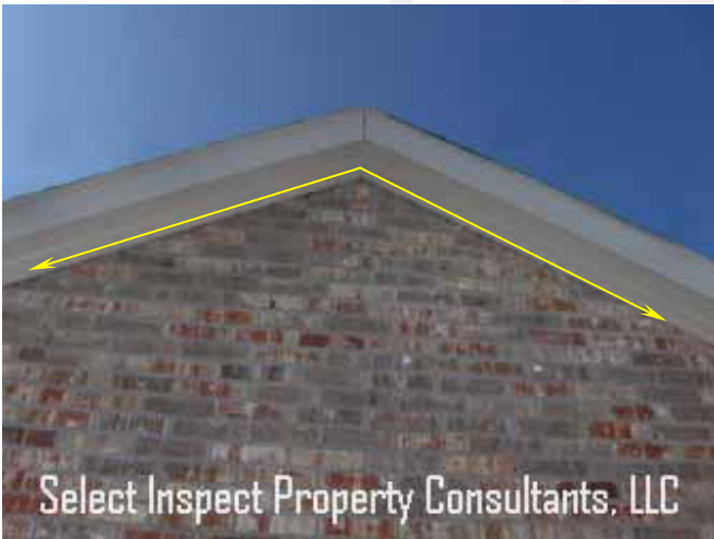
↑ short brick/openings exist; garage
