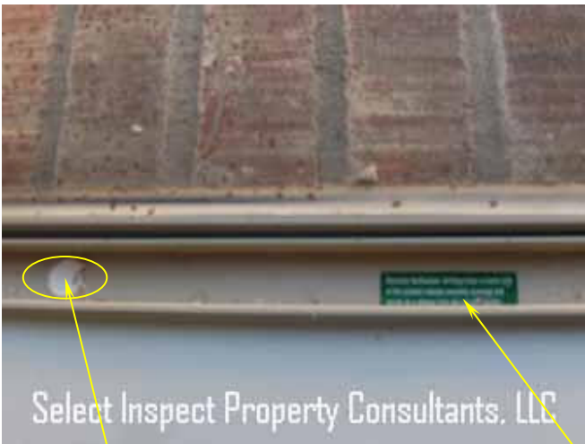
↑ Alarm holes at the lower portion of the window void manufacturer warranty; ** recommended method
