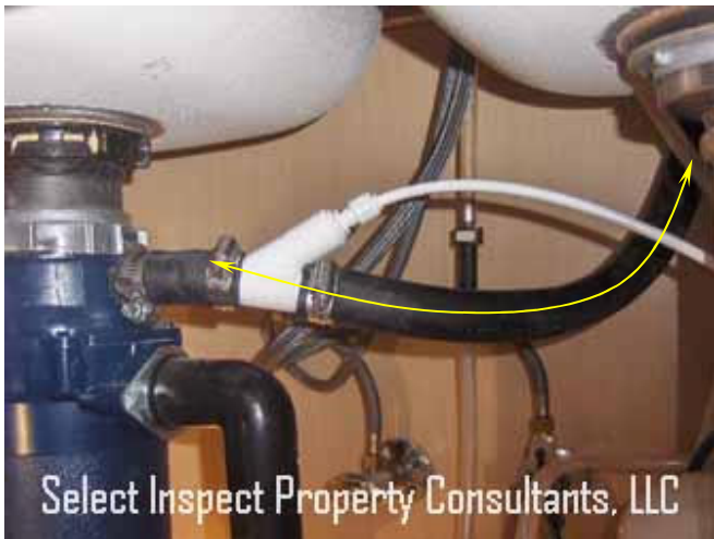
↑ drain for the dishwasher was improperly routed uphill; this should gravity drain from the backflow device
