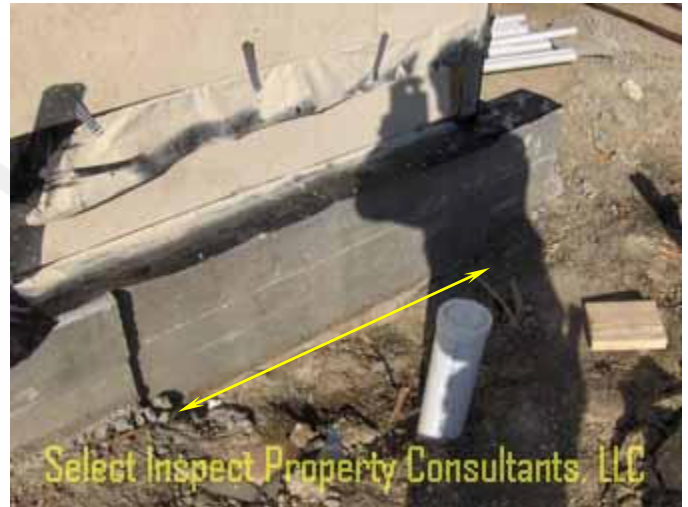
↑ form board remains at two-car garage east
