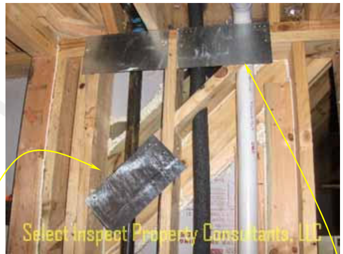
plates had been added as of Friday morning; see text above in the Interior Structure section; pg 5
