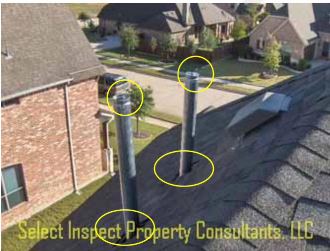
↑ flue caps & boots had been installed by Friday morning
