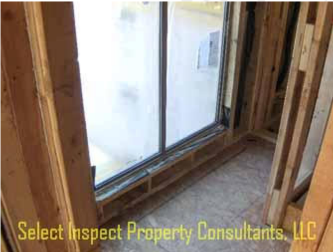
↑ low window at east bedroom closet; safety advisory, depending on intended use
