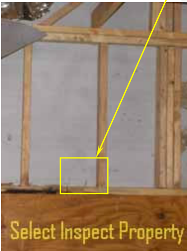
↑ close view of image above
