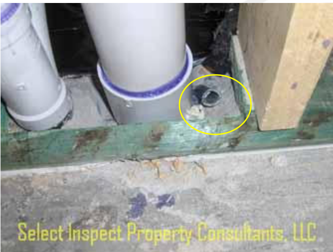
↑ hollow tube for plumbing support; example at master bathroom; may be a potential access location for termite(s) in the future.
