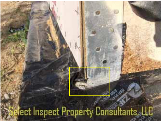
↑ tape flash improvement recommended at strap-tie holddown; southeast
