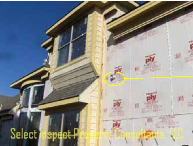
↑ tape flash & sealant incomplete at exhaust fan(s)
