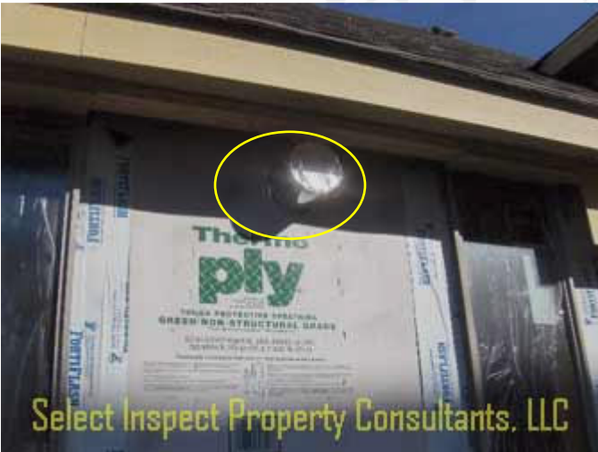
↑ kitchen vent not yet flashed/sealed during the inspection
