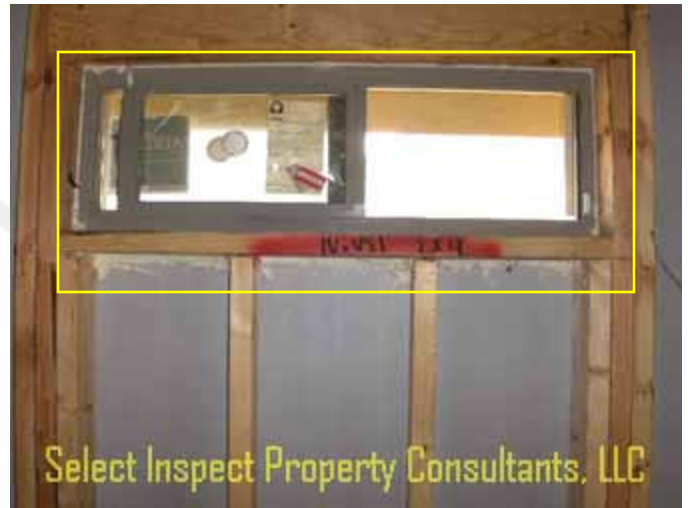
↑ sealant needed; example; at upstairs bathroom south; this window also had incomplete flashing at exterior and no visible moisture barrier * related exterior image on page 24 lower left in this report
