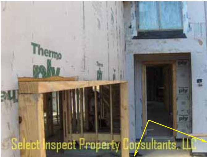
↑ forms remain at two-car garage & living room
