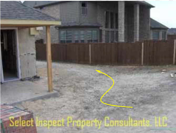
↑ swale at southwest appeared adequate
