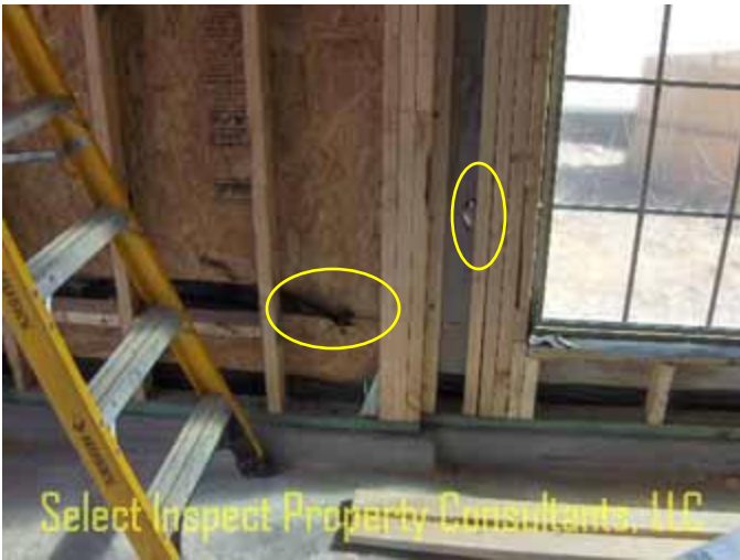
↑ sealant needed; example; at two-car garage
