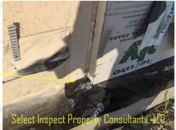
↑ tape flash improvement recommended at strap-tie holddown
