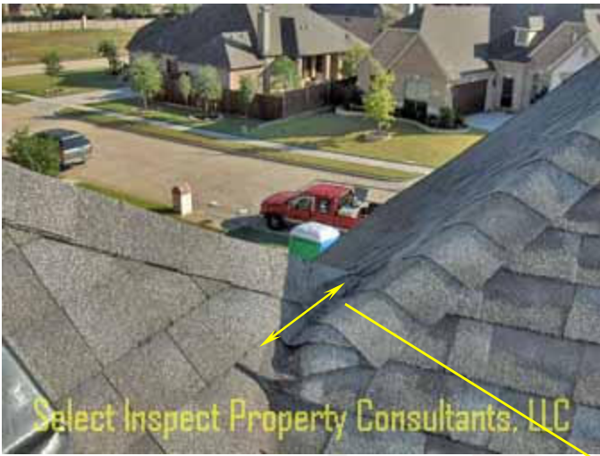
↑ inadequate slope at converging valley
