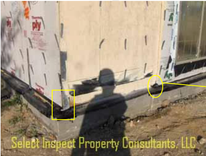
↑ tape flash improvement recommended at strap-tie holddown; southeast
