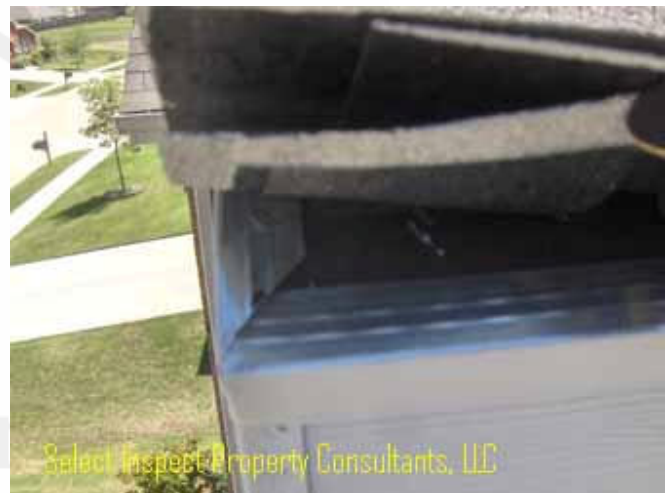
↑ unworkmanlike roof underlayment under drip edge flashing
