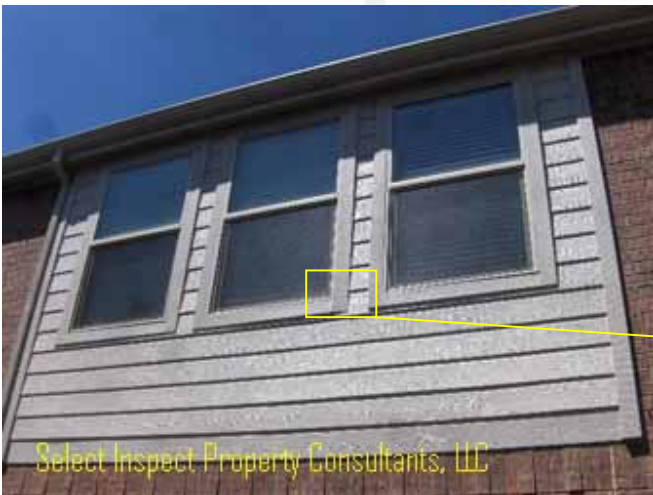
↑ unworkmanlike-uneven window trim; also reversed – inverted at all trim on this side of home.
