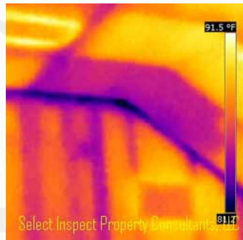
↑ Thermal imaging from square at left
