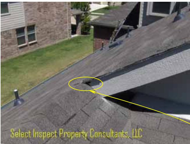
↑ unworkmanlike eave/roof connection; openings & visible decking
