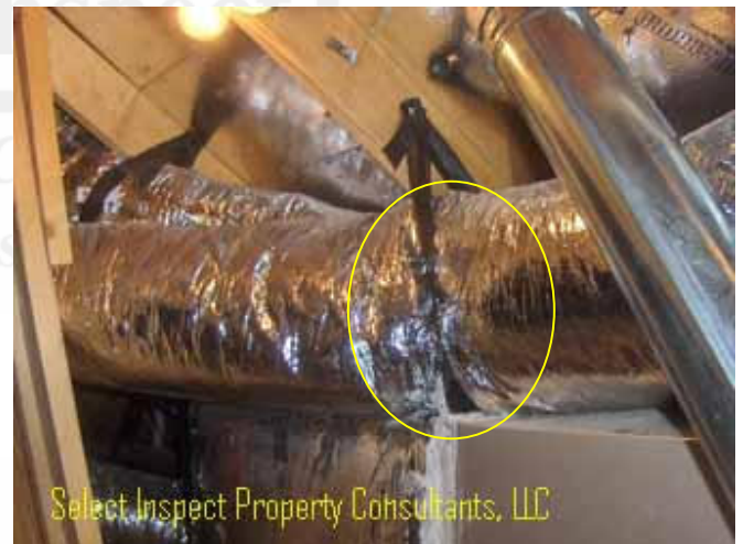
↑ crimped air ducting; example
