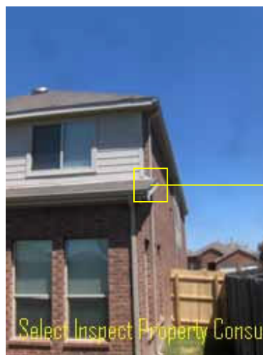
↑ short lap at drip edge flashing
