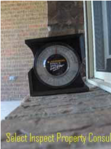
↑ brick ledge(s) had inadequate slope
