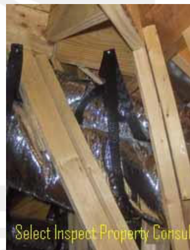
↑ crimped air ducting; example
