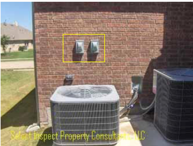
↑ incorrect location of air conditioning condenser(s) service disconnect; inadequate clearance of electrical panel for service personnel
