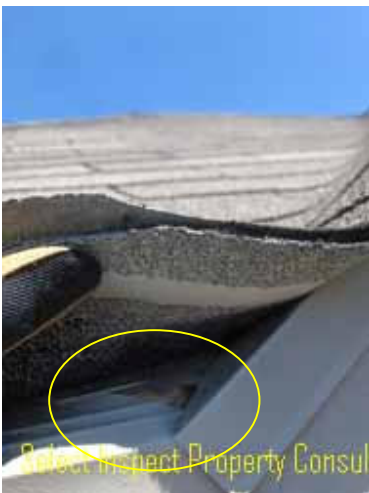
↑ deficient roof underlayment & drip edge flashing; over media room window
