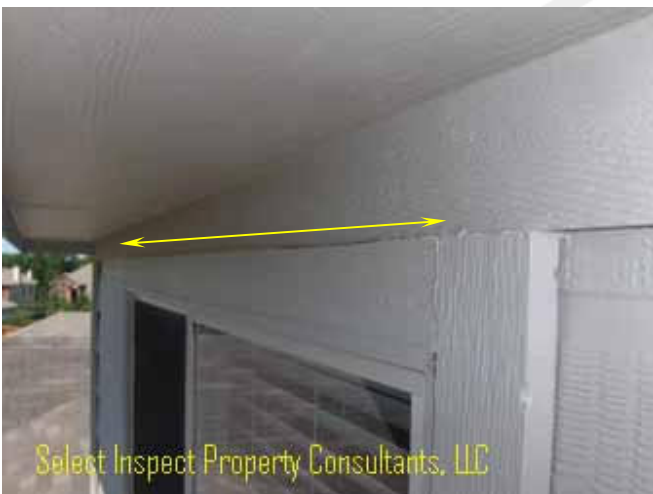
↑ gap over rear upstairs window; frieze-board & some trim here also reversed
