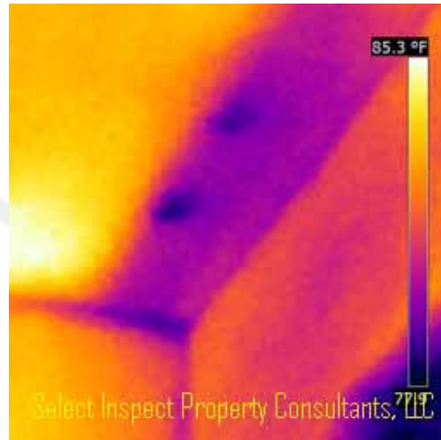
↑ Thermal imaging from square at left
