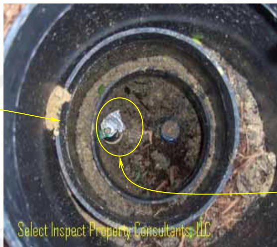
↑ pressure reducing valve had inadequate clearance from soil; Shut-off-valves require 3" clearance from soil
