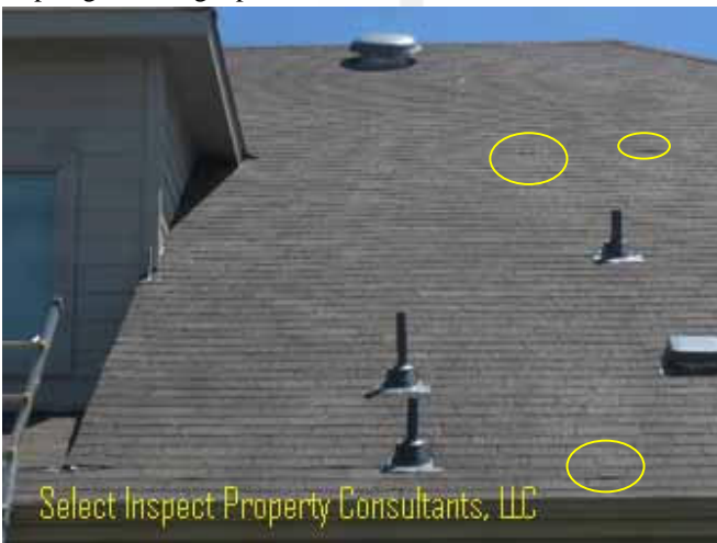
↑ Popped nail/fasteners & worn shingles at the west
