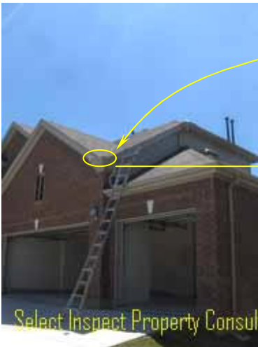
↑ short roof underlayment & short drip edge flashing lap
