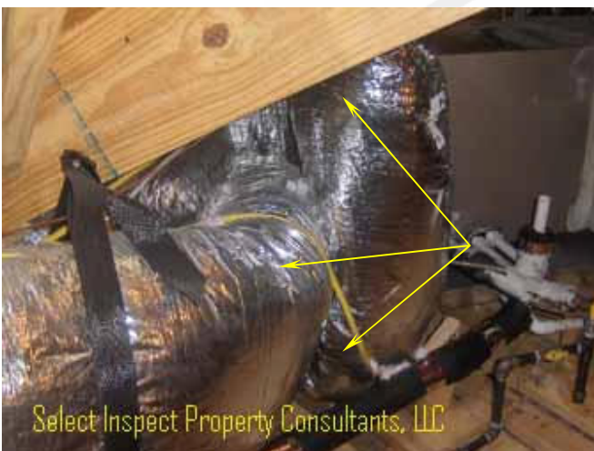
↑ crimped air ducting; example
