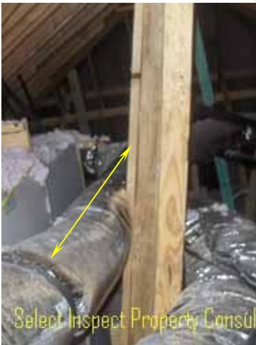
↑ crimped air ducting; example at the west side of the foyer
