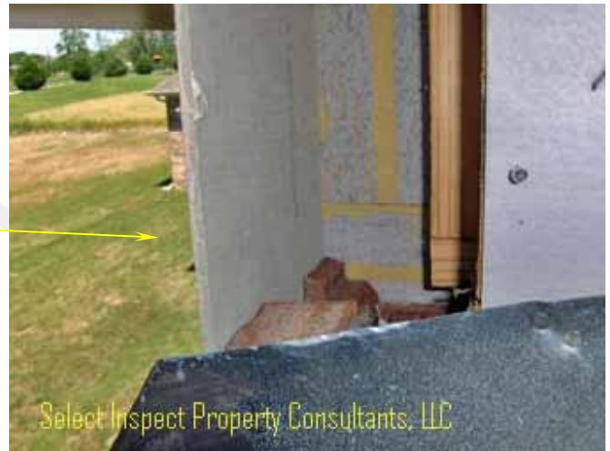
↑ close view of image at left; incomplete vapor barrier/sheathing, exposed framing; opening to wall void & attic space
