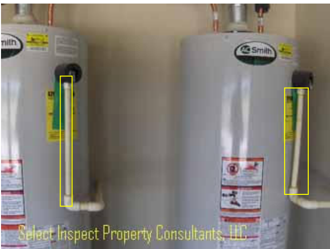
↑ water heater temperature/pressure relief piping was smaller than required by the device manufacturer
