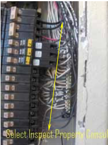
↑ paint/texture overspray in electrical cabinet
