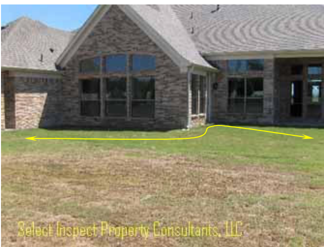
↑ marginal grading/slope
