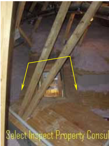
↑ there should be a minimum 24" pathway to the HVAC from the top of the access, with no gaps or obstructions; need to add appropriate decking at sides or reverse the stair/ladder
