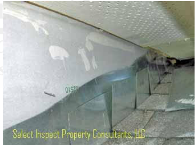
↑ close view of image above; openings & inadequate lapping of step flash; missing wall/counter flashing
