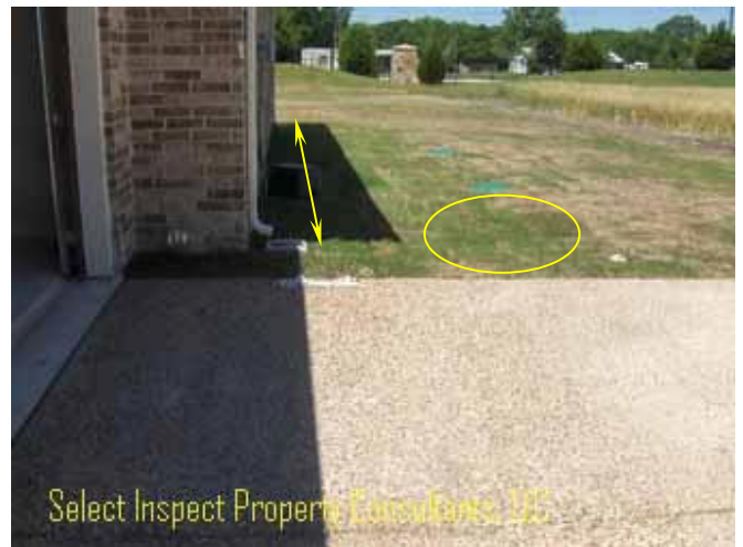
↑ marginal grading/slope & low point at soil
