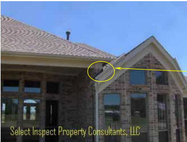
↑ incomplete wall; incomplete unworkmanlike roof & flashing; openings; moisture damage & fungus concern
