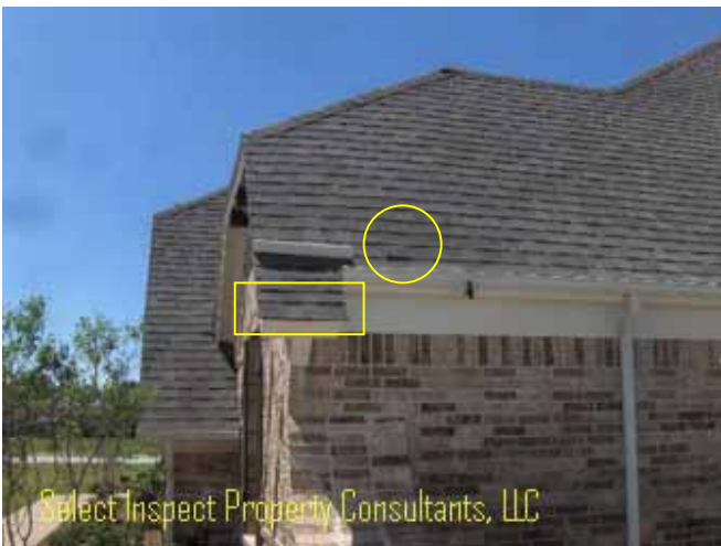
↑ example-unworkmanlike drip edge/felt; corners should have no gaps; rake (diagonal) edge & roof felt should be atop the eave (lower) edge flashing; roof underlayment should be under rake flashing. Also shown- metal protruding below shingle
