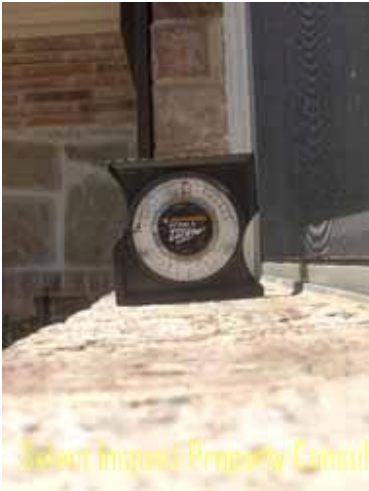
↑ brick ledge(s) had inadequate slope
