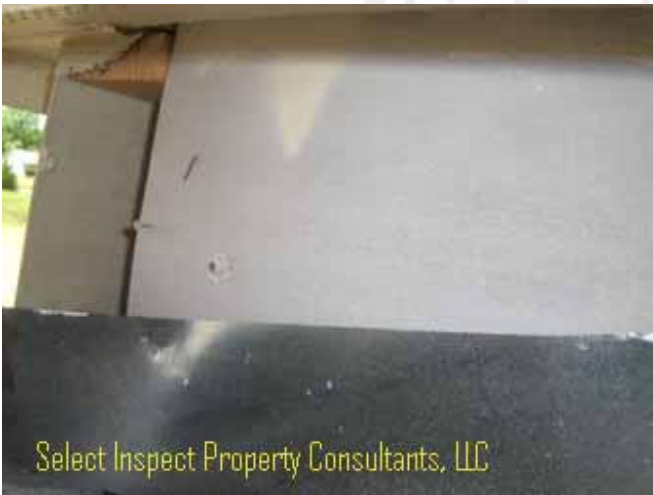
↑ close view of image above; missing siding, trim & exposed framing
