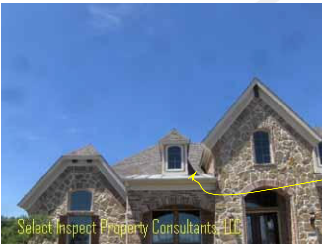
↑ opening; daylight seen from attic
