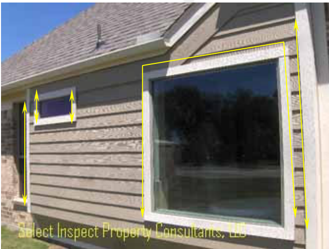
↑ trim, siding, window joints should be sealed; examples
