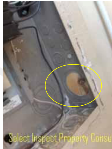
↑ missing knock-out; Deficient excess reveal exists in electrical cabinet
