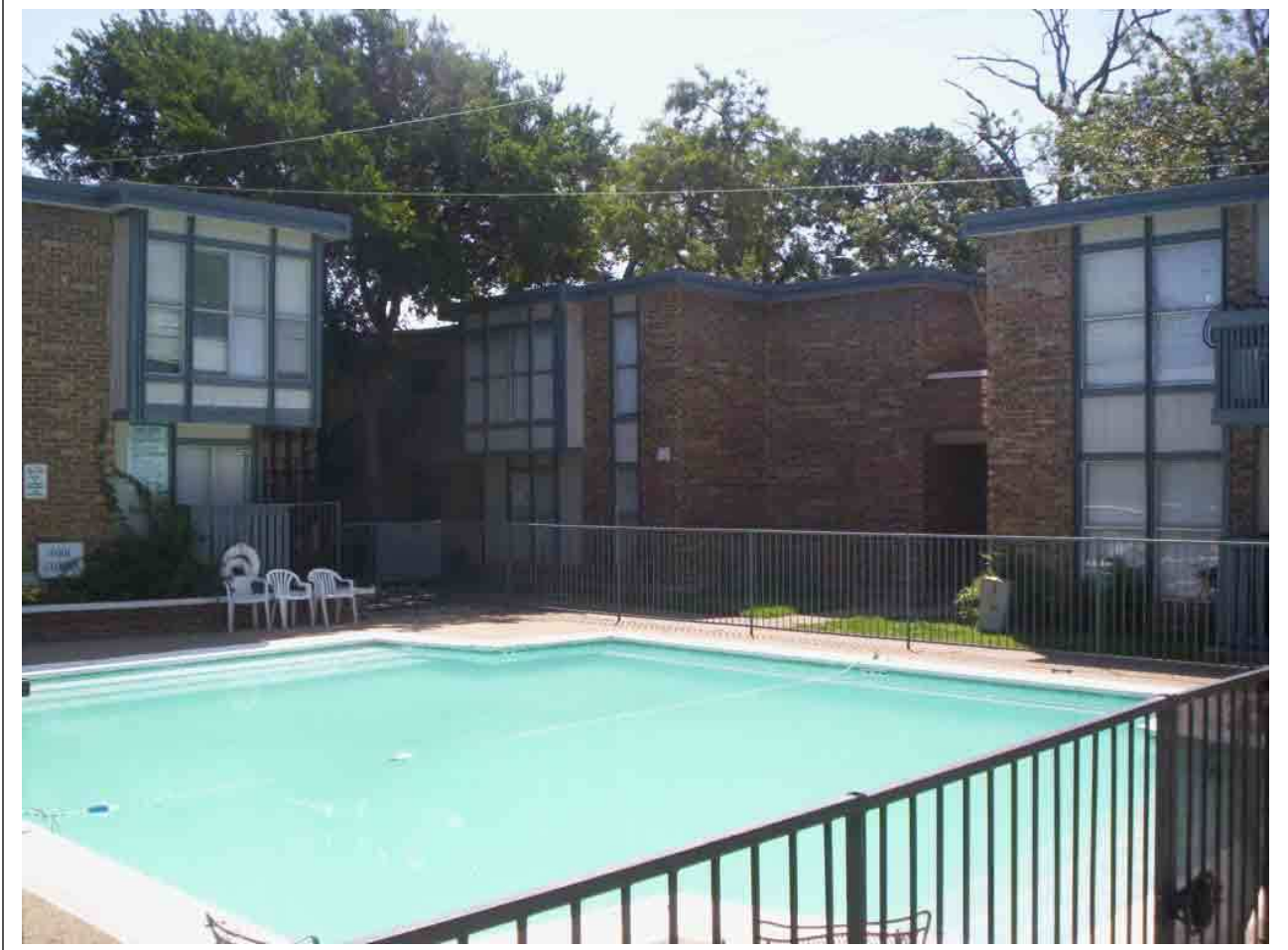
49. Comments: pool located near office- central/south area of complex
