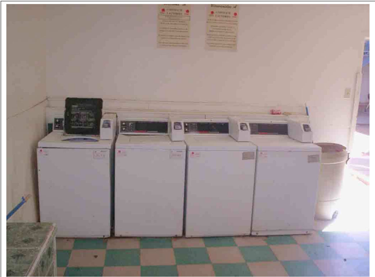
46. Comments: property has one laundry facility at south end of complex.
