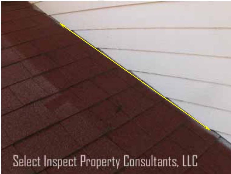
↑ low siding; prone to moisture damage; moisture damage was noted at some locations; example
