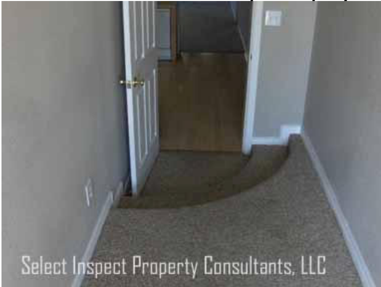
↑ steps & not wide enough doorway for handicapped access
