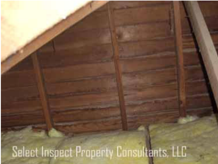
↑ example moisture intrusion in attic at gable wall siding
