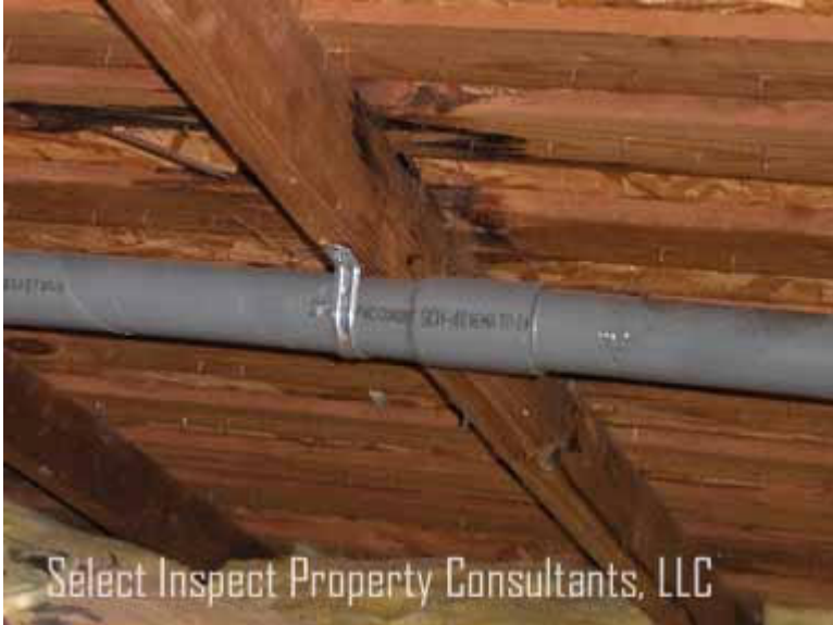
↑ example moisture intrusion in attic
