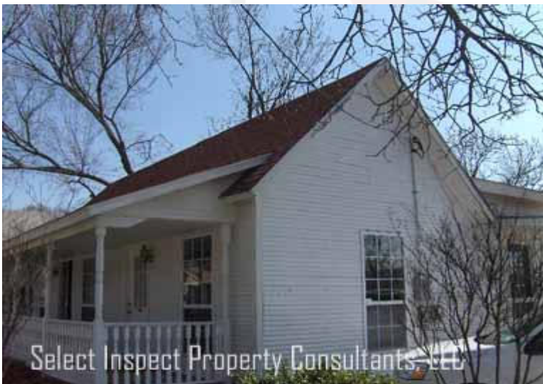
↑ service entry should not be routed through trees
