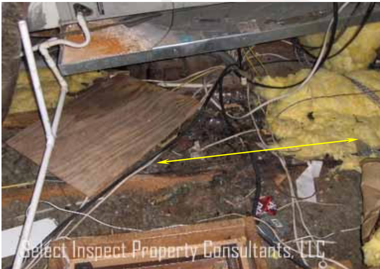
↑ fire damage at 7043 attic
