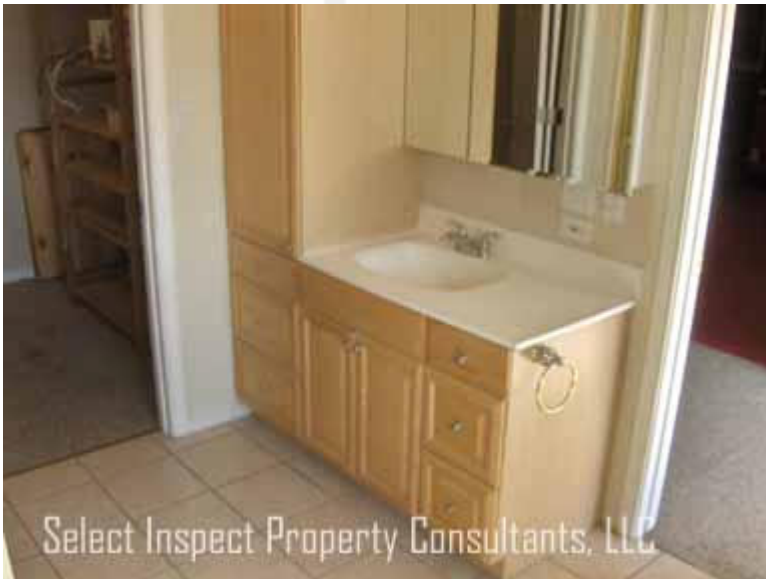
↑ sink not handicapped accessible
