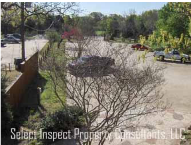
↑ inadequate handicapped parking & access
