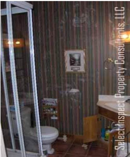
↑ toilet leaks; I turned off the water supply at this fixture; moisture damage & fungus noted below the sink
