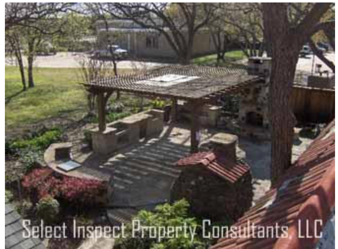
↑ outdoor showroom electrical & appliances were not tested; & were minimally inspected; I suspect you intend to update & personalize these.
