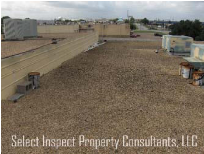
↑ shop roof; workmanlike/in good order; Monitor; provide routine service, and maintain.
