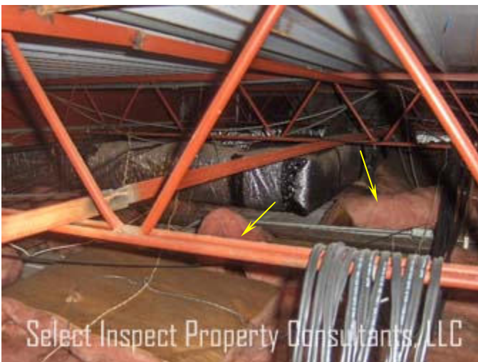
↑ insulation between levels was amiss; example
