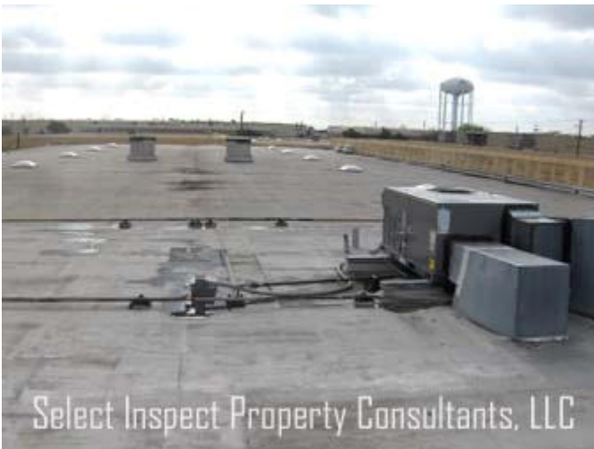
↑ warehouse roof; generally good condition, with some areas of inadequate slope
