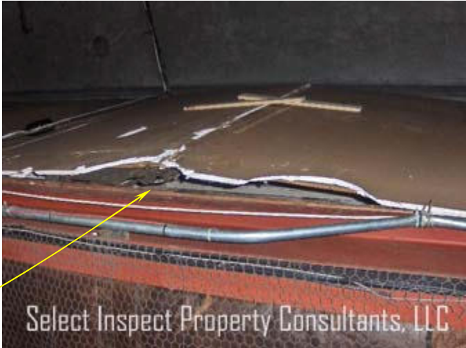
↑ unsteady/hinged wall viewed from below
