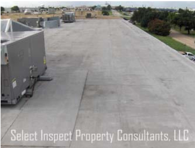
↑ office roof; workmanlike/in good order
