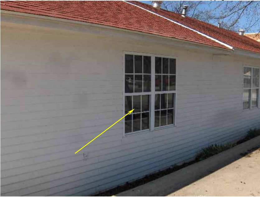
Windows seen from exterior of 7043
