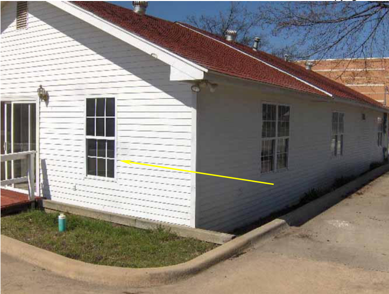
Window seen from exterior of 7043
